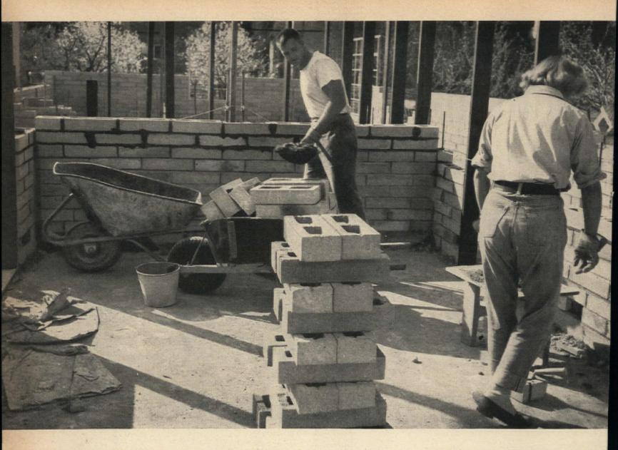
For an owner-built house, concrete brick was a wise choice of material since it is thick enough to require no inside wall construction, and because the small units are relatively easy to handle. When they were delivered, they were & it in piles near the spots where they were to be used—a bit of foresight which saved the Booths both time and labor
