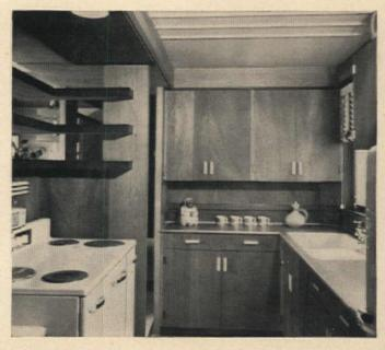
The kitchen is minute, but so well planned that it has plenty of counter and cupboard space—and enough room for an automatic washing machine. For economy in building, it backs up to the bath
