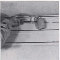
For small areas, doors, woodwork, and window trim where the regular rollers won't fit, a special 3or 4-in. roller is handy and speeds up the work
