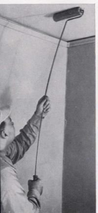
A long-handled roller, or a regular roller with a long handle improvised and fastened securely to the short handle, will do away with much of the ladder or scaffold work on ceilings and high parts of walls. It will reach behind radiators too. Painting or varnishing floors, the same long-handled roller saves backaches
