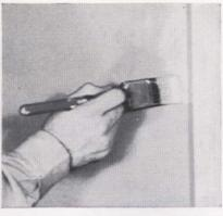
Around woodwork, ceiling line, and corners, where you can't work with a roller, paint a strip with small brush. Do small section at a time so it will be wet when you roll up to it, and won't show a lap mark
