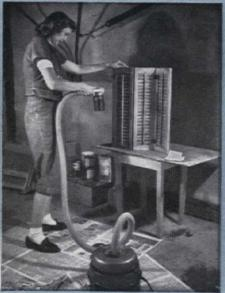
First coat of finish is applied, then assemble shutters with hinges and complete finish. Paint or shellac can be sprayed with gun or vacuum attachment
