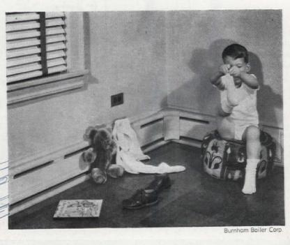
Unobtrusive baseboard convectors spread the heat at floor level along outside walls. This one has fins to heat the air as it passes in bottom and out top
