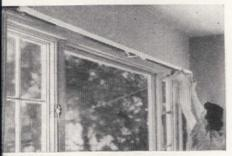
Insert rod in brackets. Long rod such as this one requires a center support firmly screwed to window frame
