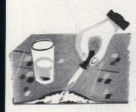
A flat board, a breadboard is fine for job, placed over repair and held down by a heavy weight overnight, is sufficient to hold linoleum permanently
