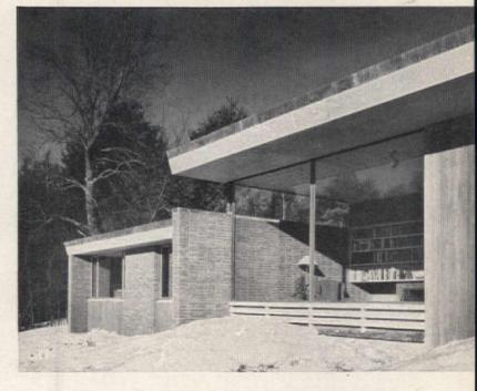
House combats variations of New England climate by use of solid brick walls, large glass areas with heavy overhanging eaves for solar control. Roof is flat, built-up; eave flashing provides for one inch of water for summer cooling
