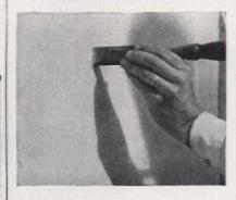
n walls of plaster or wallboard, start the cut with a chisel. Start with a drill in wood walls. Use a cold chisel to cut brick or concrete walls
