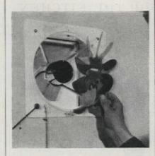
Wiring within the wall should be done by an electrician. The unit shown was altered for connection by a wall plug. Hook up outside trap or louvered door, complete wiring, put fan on shaft, install interior grill, and check operation of the complete unit. Some built-in kitchen ventilator fans require circular openings, but the one shown needed square cuts for both inside and outside walls
