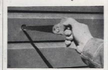
ail provides a base for laying out pattern of outside cut. Complete opening in wood or masonry walls as indicated for interior walls above
