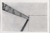
Jut opening in interior wall with key-U hole saw; remove insulation. Drive a center nail through outside wall
