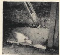
letail of top of adjustable bearing post shows built-in jack feature which makes job so much simpler. Cement mix for concrete is I part cement, 2 parts sand, and 3 parts gravel. Form can be built simply of light wood and removed when the base has set-in about three days
