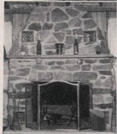
Grilles for upper warm-air outlets have been set in place, stonework from the mantel to ceiling is completed. Logs are laid and ready to be lighted PICK INSULATION WITH FIRE IN YOUR EYE!
