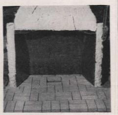
A glance within the cabin shows insulation completely covering unit. Hearth has been laid and is ready for fire-clay mortar which will go between cracks in bricks
