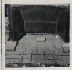
Wooden form was built into which concrete was poured-note crisscross of steel rein forcing rods and metal fram for ash dump in background
