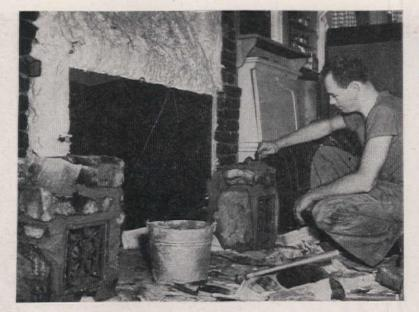
Meanwhile, within cabin, galvanized air ducts have been attached to top outlets of heat circulator. Heat cast off by burning logs will rise through these ducts and flow into room. Fireplace is to be of stone, and here Bill is constructing stone piers in the base of which he has inserted a grille. This, and a similar grille on the other side of the opening, will draw cold air from floor into warm-air circulator
