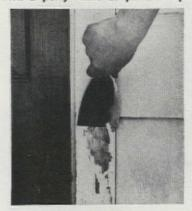
Go over rough spots with No.  $1\frac{1}{2}$  sandpaper before applying any paint. Also, let wood dry thoroughly if it is wet
