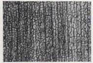
This surface was painted when the wood was wet, causing blisters. Blisters must be broken and paint removed
