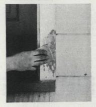
When paint has been removed to the bare wood, bare spots should be given prime coat before proceeding
