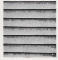
Cheap paint cracks all the way to the wood. Moisture finds its way behind the film, eventually, and scaling occurs
