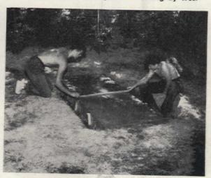
When the form is packed with cement, the surface is finished off by sliding a straight board along it, pushing off excess, and filling in depressions
