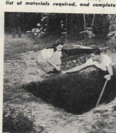
The pit is now below frost level, and ready for the three cubic yards of cinders required to provide drainage and to prevent heaving by frost
