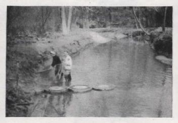
The heavy grindstones were rolled and pried into place with long bars made of small trees. This shows one tier in place and a start being made on the second
