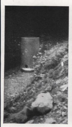
This is the drain water tile tank in place 13ft. below the spring where it bubbled up out of the hillside
