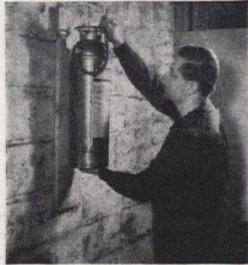
Grip nozzle of soda-acid or foam unit in lifting from wall bracket
