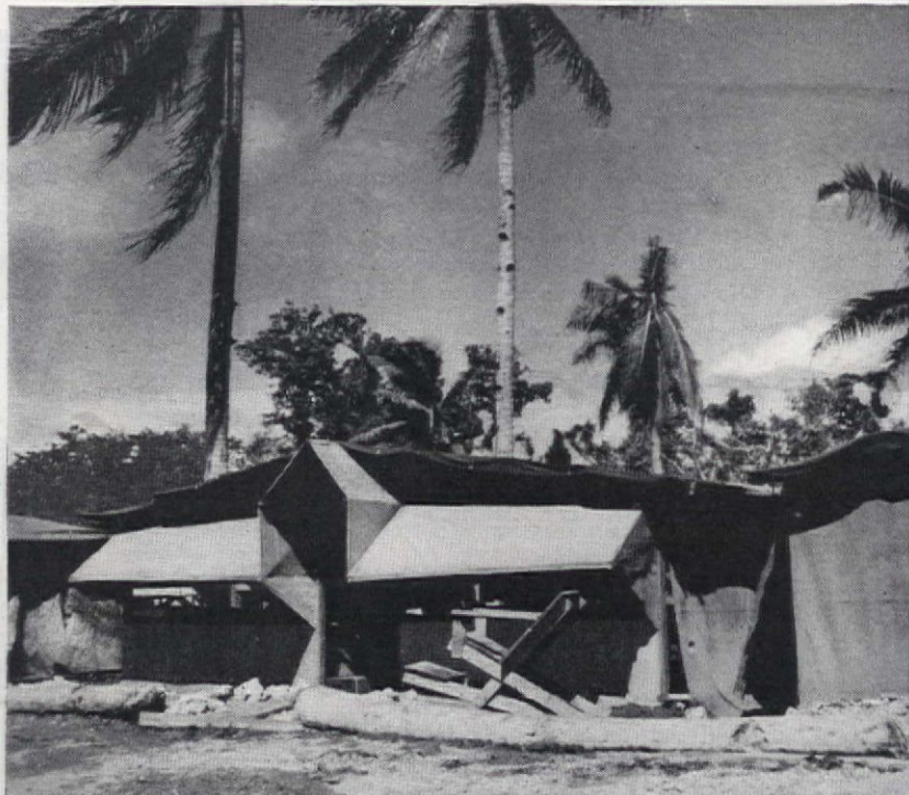
Marine flight plane mechanics built ingenious house of ponchos, palm logs and scrap canvas—the last word in functional design
