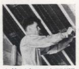
And here's how neatly KIMSUL is installed in sloping roofs. Stays put, too, once properly installed. Rows of strong stitching run through KIMSUL blanket, prevent sagging, sifting, settling.
