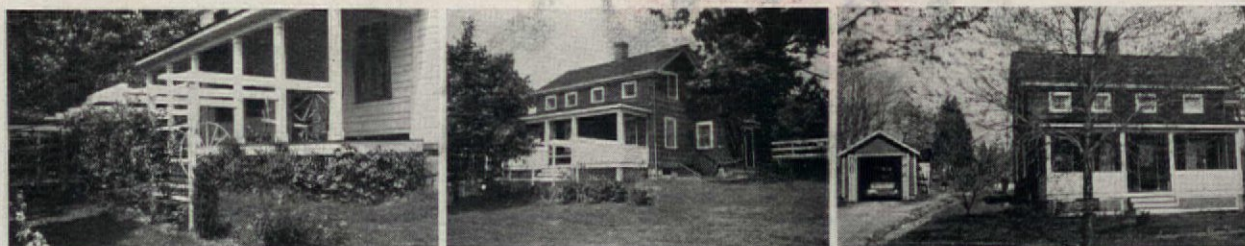
A brown mess of a house when we found it (far right), "Westlawn" had sound structure but little interest. A front arbor for trailing Dorothy Perkins roses, new flower beds, new farmhouse fencing, wagon wheels for step railings, and the place began to "pick up"
