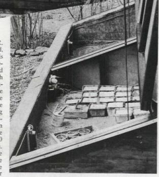
Almost human in its operation. Thermostats control the furnace-damper motors (on garage wall), which raise and lower the sash
