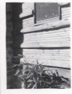
Wood board or block cabin construction. Half logs at intervals vary exterior treatment
