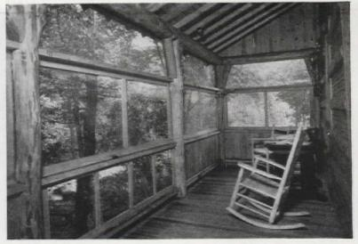
The walls are constructed of 2x4" boards, varied by round logs. The boards are chamfered on the outside, beaded on the inside face
