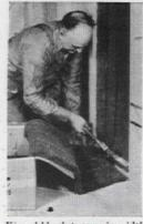
Kimsul blankets come in widths which exactly fit between stand-ard studding – save cutting and measuring on the job.
