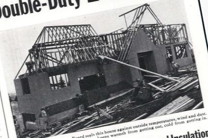
Fir-Tex Firkote Sheathing Board seals this house against outside temperatures, wind and dust.
