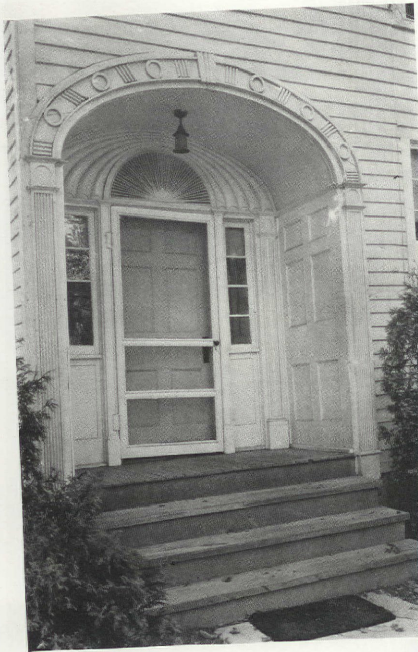
Two beautiful doors on early Ohio homes. Adam design, as interpreted by a local carpenter, on the doorway of the old dining hall of Western Reserve College in Hudson (left). The doorway of the Singletary House, in Streetsboro, bears much relation to it. These, and all photographs, described fully in text
