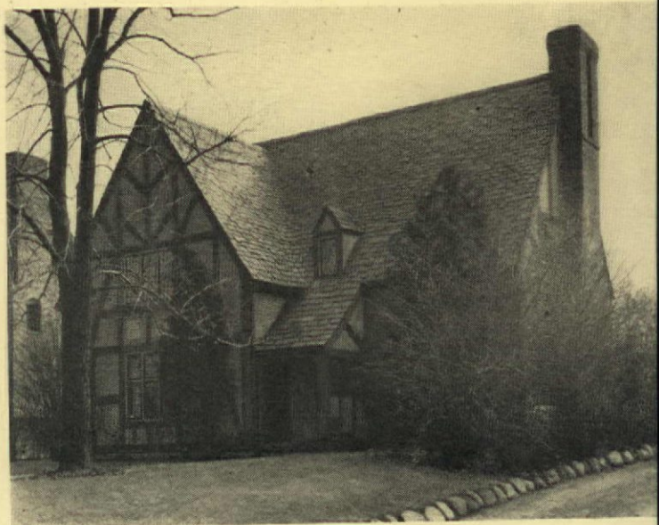
The gabled English house, like Mrs. Howard L. Hyde's, vitalized our earliest American homes. Note the high roof, decorative half-timbering of stucco walls, tiny dormer window
