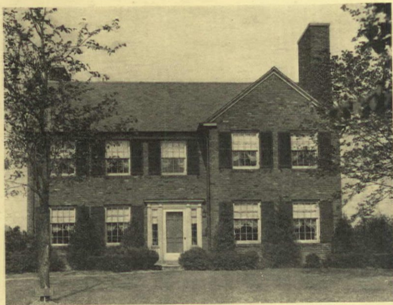
Warm brick walls, massive end chimney, pedimented front section, characterize the dignified residence of Mrs. J. F. Holihan. White trim classic portal with sidelights provides an austere polish
