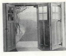
Third is the "Folding S ing" garage door, desig for openings with th four, five, or six door equal width. With this section can be opened be used as a passage when it is needed, with opening the entire door
