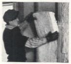
J-M Home Insulation in "batts" for new houses or "blown" in walls of existing homes. Keeps rooms up to 15° cooler in summer, cuts winter fuel bills up to 30%.
