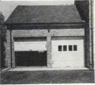
Illustrated is the so-called "Ro up" garage door. The door ro on vertical tracks and rests on ho izontal tracks when fully opene The necessary hardware is i side, away from moisture. is operated from the inside an automatic spring trip, and cord is provided to bring t door down within easy rea
