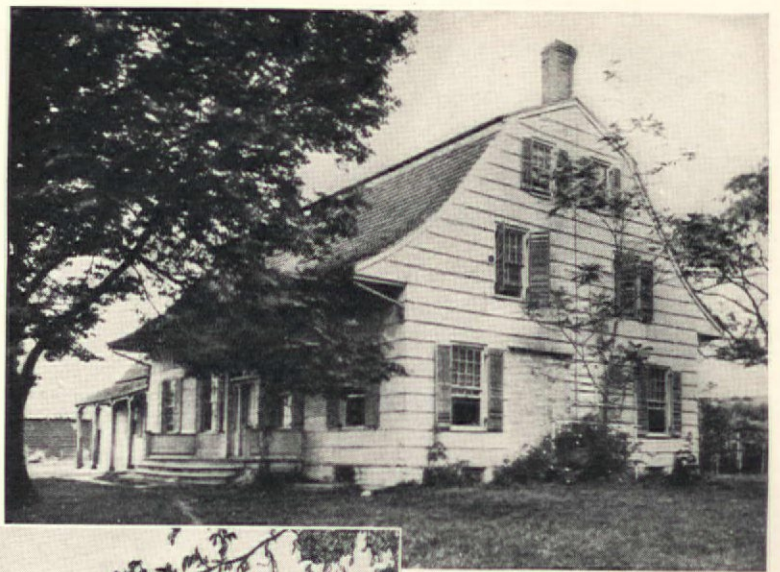
Truly Dutch Colonial. Notice the graceful roof slopes. The porch and dormer are later additions to this house and are out of character with the rest of the building. (Courtesy of Pencil Points. Photo by K. Clark)
