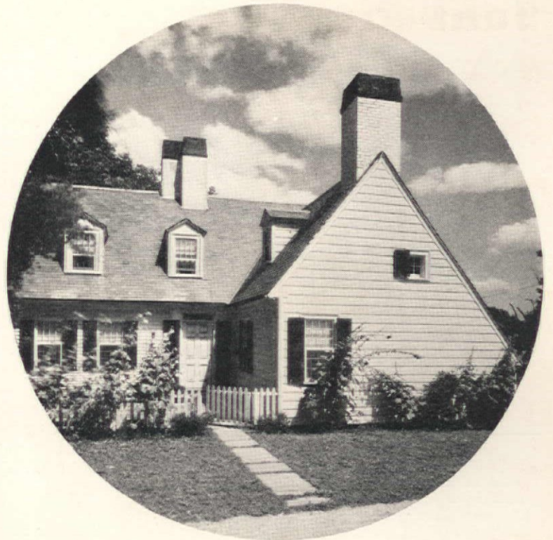
This house in Brookline, Mass., won the Better Homes in America Gold Medal for 1932. Architect, Royal Barry Wills. Painted with Cabot's DOUBLE-WHITE
