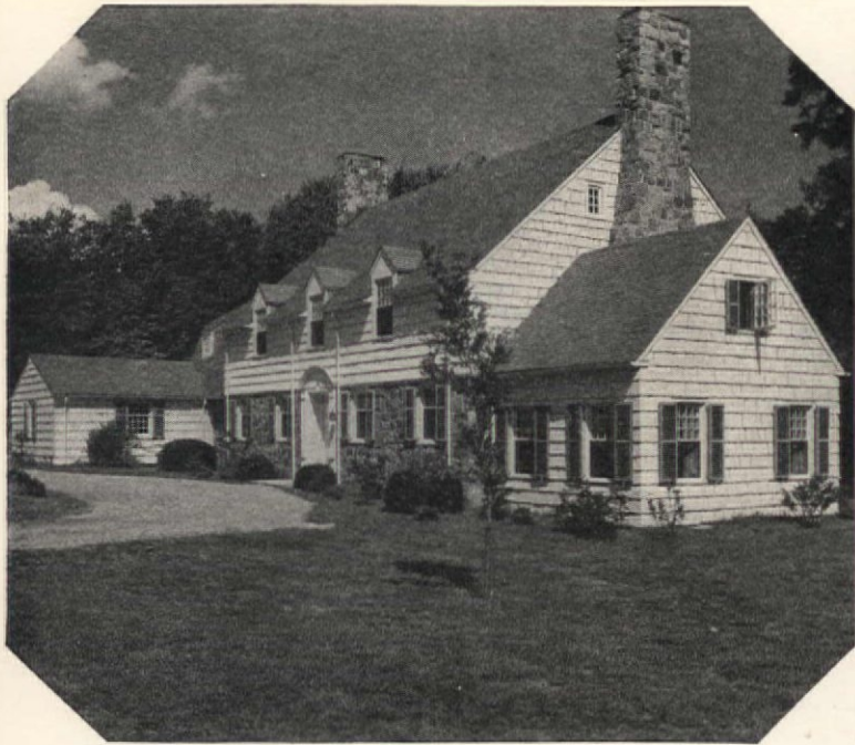
House in Knoxville, Tenn. Architects, Baumann & Baumann, Knoxville. Finished with Cabot's Old Virginia White and Cabot's Green Gloss Collopakes. Insulated against summer heat and winter cold with Cabot's Quilt.
