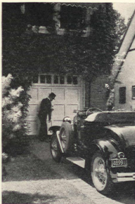
In this type of overhead door the door itself is divided into four equal sections which are hinged horizontally. (Barber-Colman Company)
