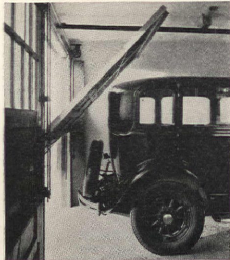
These garage doors are raised to the ceiling and slide on an overhead trolley with ball bearings. (Coburn Trolley Track Mfg. Company)
