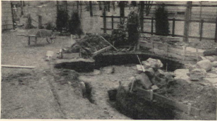
One: The earth sides as part of the form for concrete
