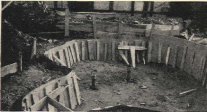
Two: Linoleum braced with wood making the concrete form
