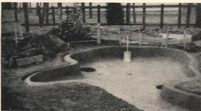
Three: Concrete poured and form removed
