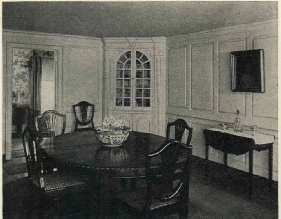
H. W. Rowe Associates, architects
