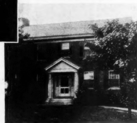
True to its name, the Cambridge presents the beauty and inviting aspects of the Colonial type home. A simple, liveable home. Shown in detail in "Beauty in Brick".
