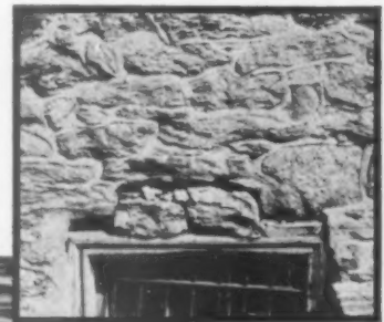
The masonry over doors and windows must be supported on suitable beams or lintels or on carefully constructed arches as shown below to prevent the settling and cracking which occurs if the masonry is allowed to rest on the wood frame of the window or door. At the right is seen what happens when the precautions are not taken
