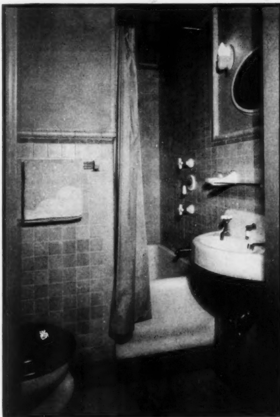
Even where space is at a premium a compact bathroom such as this may be ingeniously installed, for bathroom fixtures are now designed in all sizes and styles to meet all conditions. (Courtesy of the Kohler Co.)
