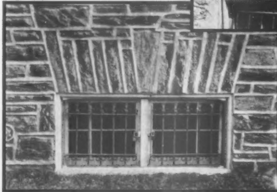
The masonry over doors and windows must be supported on suitable beams or lintels or on carefully constructed arches as shown below to prevent the settling and cracking which occurs if the masonry is allowed to rest on the wood frame of the window or door. At the right is seen what happens when the precautions are not taken
