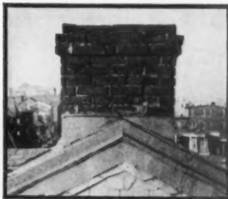
Chimneys receive the full force of storms, the scorching sun, the hot gases from within the chimney, and the disrupting action of frost. Their tops must be protected by a solid stone or cement cap, as below, which will prevent water from saturating the chimney, freezing and expanding and causing the damage seen at the left
