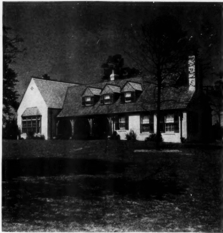
A charming new home in Mobile, Ala., designed by George B. Rogers, Architect. Shingles and trim are stained with Cabot's famous Gray Creosote Shingle and Wood Stains.
