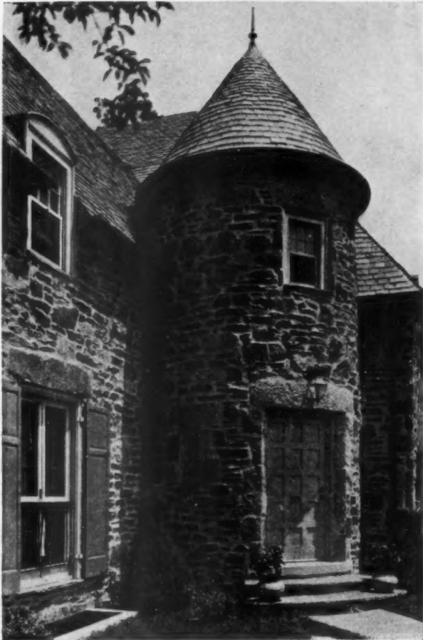
A charming residence of the Norman type, completely equipped with Sargent Hardware, O. Eugene Adams, architect, Baltimore, Md.
