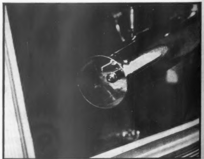
The "business end" of a "gun" type of burner showing the interior nozzle which atomizes the oil as it is forced into the boiler. The electrical poles where the igniting spark is made are at the end of the nozzle
