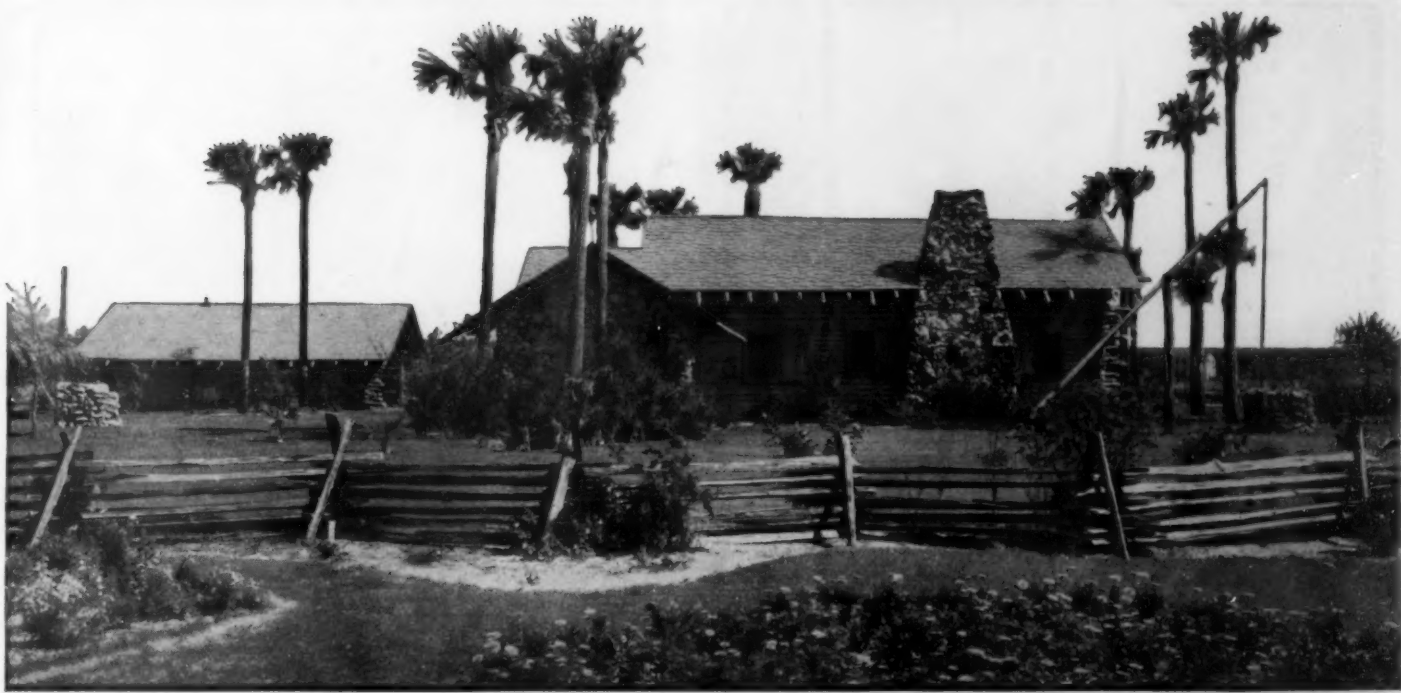
This house built by Mr. and Mrs. H. Carl Dann at Mount Plymouth, Florida, is of pine logs and stone such as the pioneers built sixty years ago. The split rail fence enclosing the attractively landscaped grounds was brought from a backwoods farm twenty miles away
