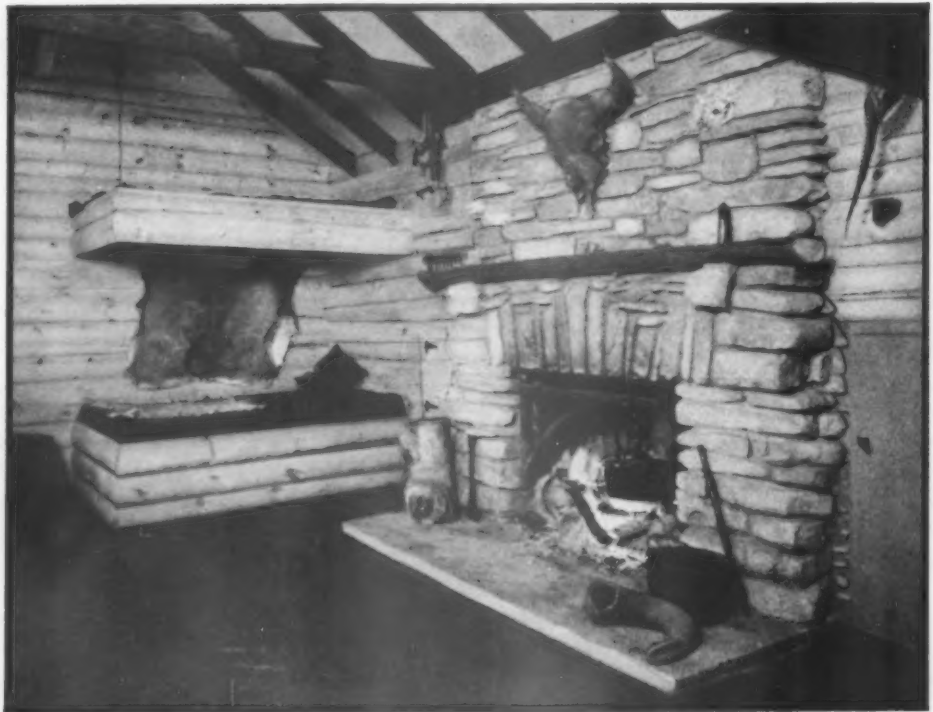
Log siding was used on the interior of this house located in the Minnesota River Valley near Minneapolis. W. H. Tusler is the owner and architect. (Photograph by courtesy of Shevlin, Carpenter & Clarke Co.)
