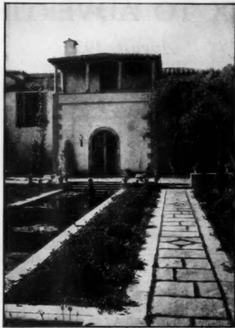
All the beauty of natural flagstones is found in these hand-made slabs of concrete
