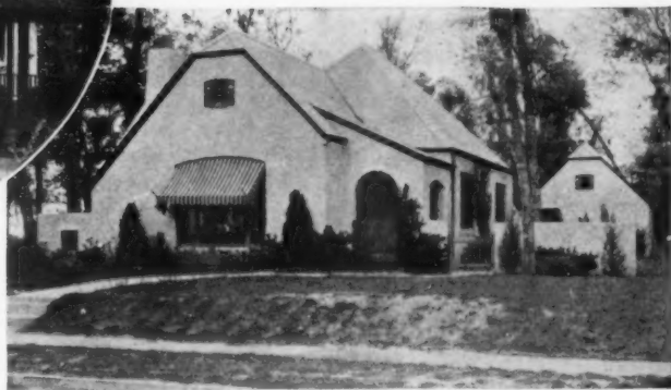
Residence of Dr. Walter Dickson, Houston, Texas. G.O. Thiel, Architect. Concrete masonry walls, faced with gray portland cement stucco.
