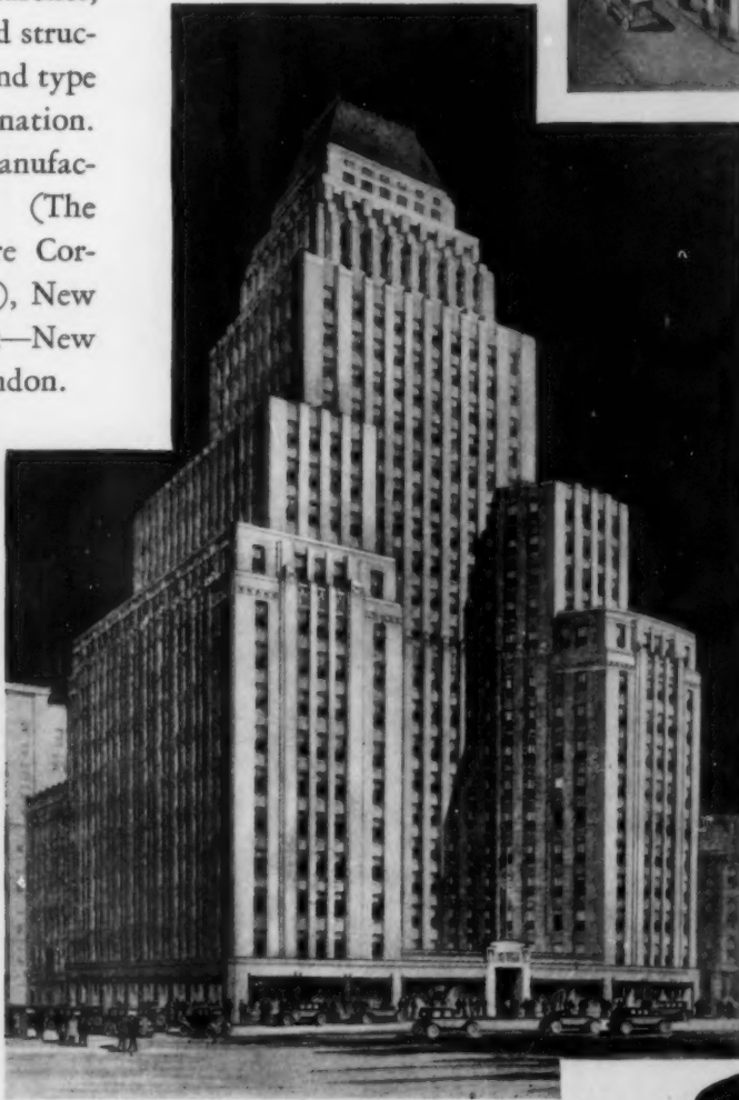
The UNITED SHOE MACHINERY Bldg. Architects Parker, Thomas & Rice, Boston, Mass. Associate Architect Henry Bailey Alden, Boston, Mass. Contractors Geo. A. Fuller Company, Boston, Mass. RUSSWIN Dealer Chandler & Barber Company, Boston, Mass.
