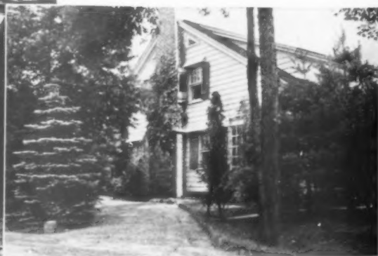
The architect, Arthur T. Remick, New York, employed the same rugged lumber in the beautiful new home of Arthur W. Wood, Westchester, N.Y.
