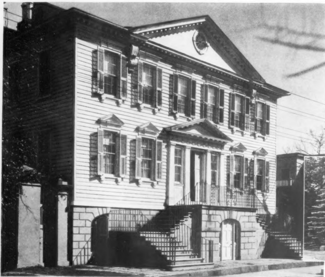
Tidewater Red Cypress was used throughout the Gibbs Home in Charleston, S. C. . . . Built before 1800, it is sound as a dollar today.
