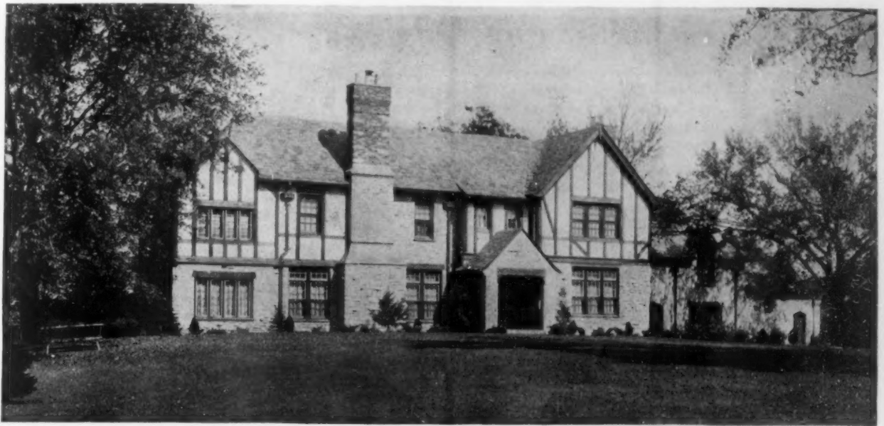
Residence of Howard Swallow, Esq., Danville, Ill. Lewis and Dougherty, Architects. Concrete masonry walls and partitions; lower story faced with stone; upper story, half timbered portland cement stucco.
