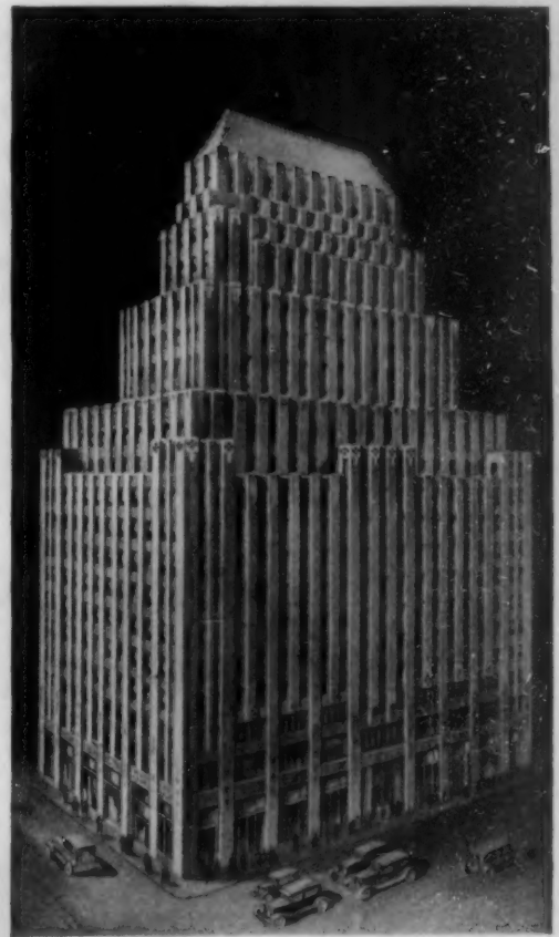
The ROLLINS Bldg. Architects Thomas M. James Co., Boston, Mass. Contractors Thompson-Starrett Co., New York City RUSSWIN Dealer Chandler & Barber Company, Boston, Mass.
