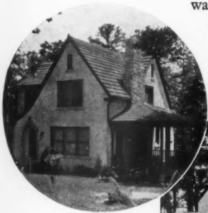
Residence of Harry Angle, Chattanooga, Tenn. Percy Shepherd and Chas. B. Sears, Architects. Concrete masonry walls faced with buff portland cement stucco.
