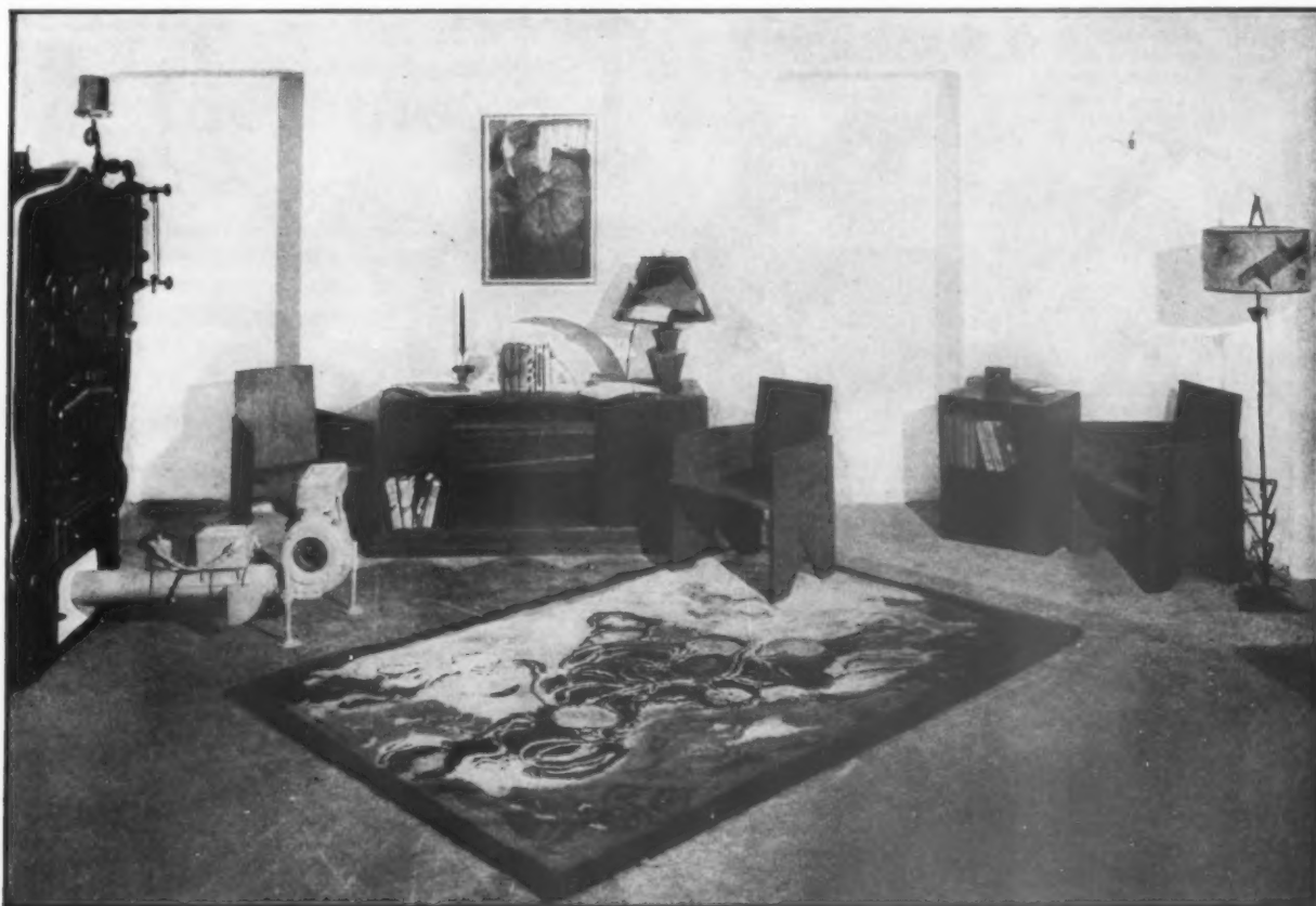
The oil burner, eliminating the dirt and dust of coal, makes possible the utilization of space in the basement for reading or recreation rooms
