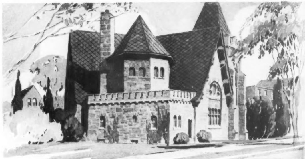
How perfectly this attractive roof of J-M Mottled Gray Hexagonal Asbestos Shingles blends with the architecture of this Toledo, Ohio, Church. Schools, institutions, churches — as well as residences find permanent roofing beauty and protection in J-M Shingles.
