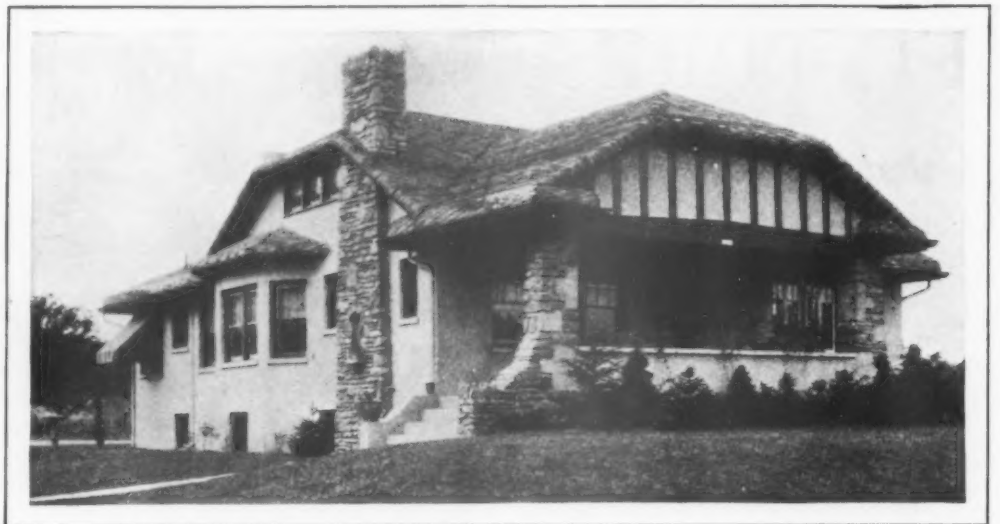
Home of John Clopmeyer, Cincinnati. Concrete masonry walls, with portland cement stucco exterior. Designed by the owner.
