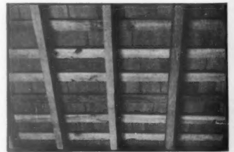
This is what the underside of a properly constructed shingle roof looks like
