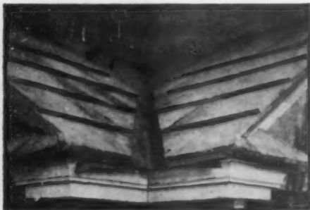
Corner of a well-constructed shingle roof. See text for details
