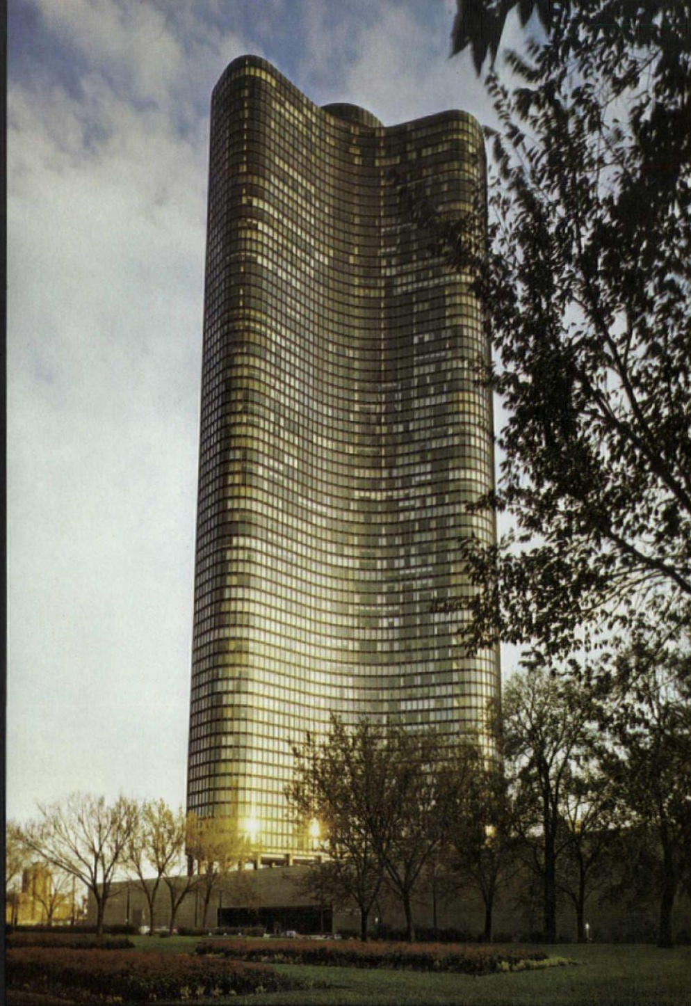
LAKE POINT TOWER, Chicago, Illinois/Architect: Schipporeit-Heinrich/ General Contractor: Crane Construction Co./ Glazing Sub-Contractor: National-Hamilton, Div. of Bienenfeld Glass Corp. 1" Polarpane glazing manufactured by Polarpane Corporation
