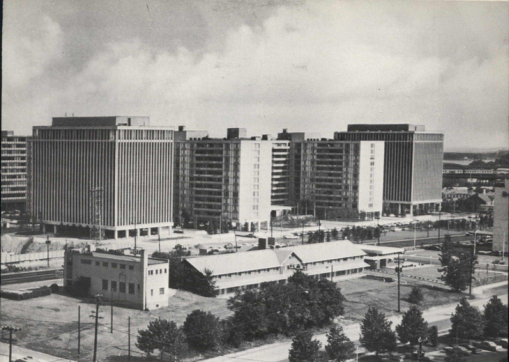
Ceco Steelform Service for 790,000 sq ft of monolithic concrete joist construction 12,700 tons of Ceco-fabricated Reinforcing Steel 480,000 sq ft of Cecocolor Anodized Aluminum Windows and Curtainwalls
