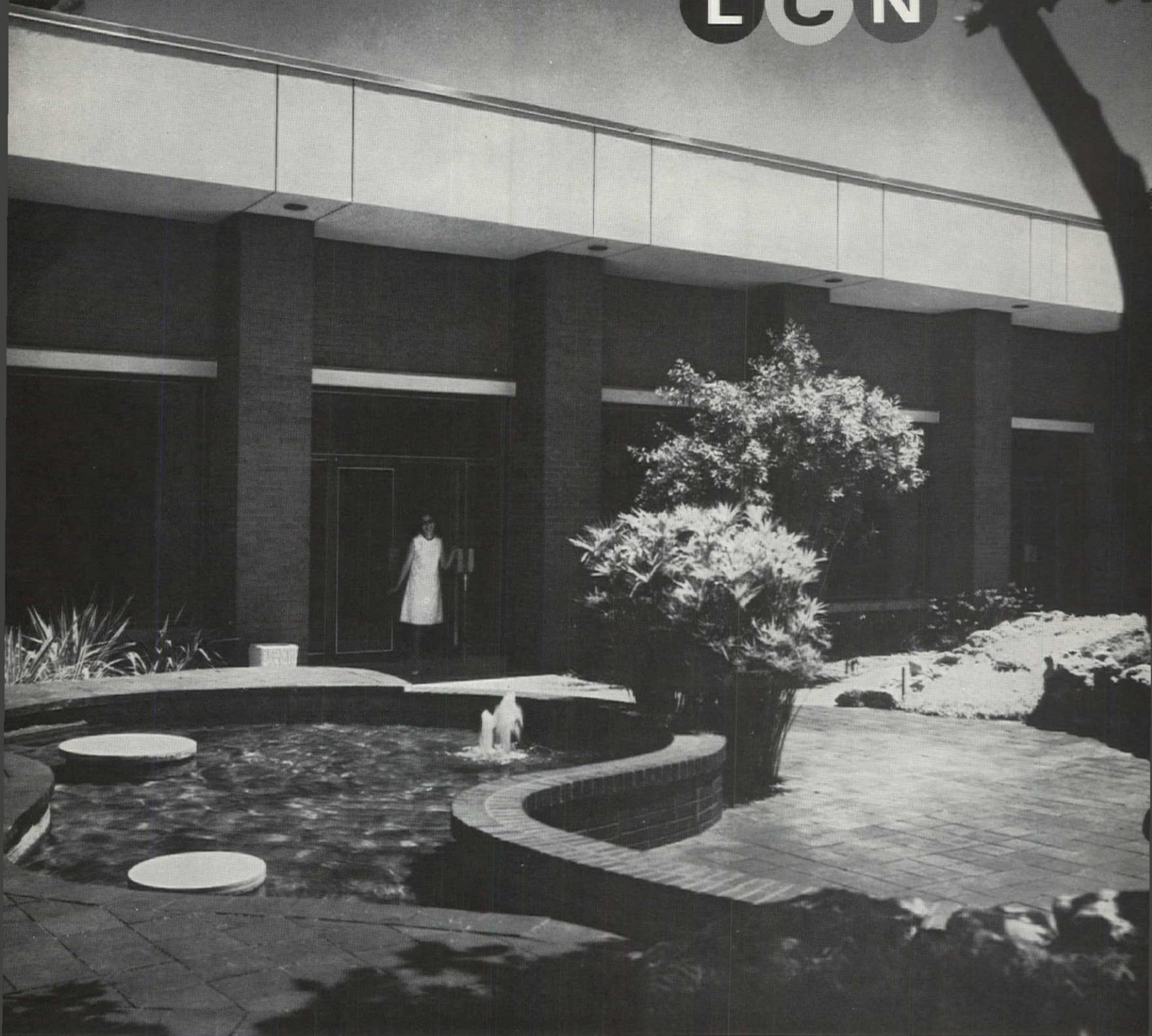
Overseas Operating Center, American Telephone and Telegraph Company—Long Lines Department, Jacksonville, Florida. Reynolds, Smith and Hills, Architects—Engineers—Planners; Jacksonville.
