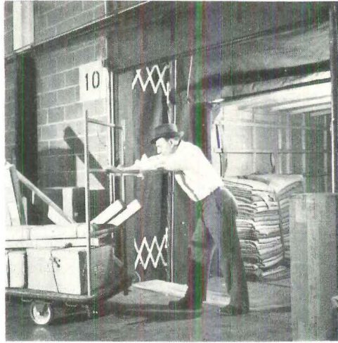
Merchandise is unloaded on wheeled "float" which rolls it through building
