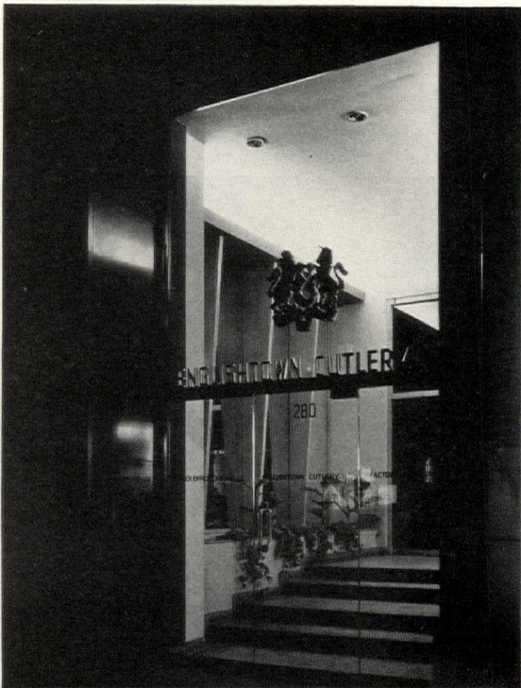
ENTRANCE STAIRS ARE DISTRIBUTED IN THREE RUNS TO EASE THE 3 FT. RISE FROM STREET LEVEL
