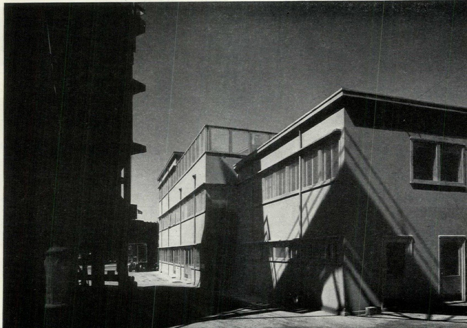
GLAZED SCREENS PROTECT EMPLOYEES' SUN DECK FROM SHARP BAY WINDS. WINDOWS ARE SEALED AGAINST DUST, OPEN ONLY FOR CLEANING
