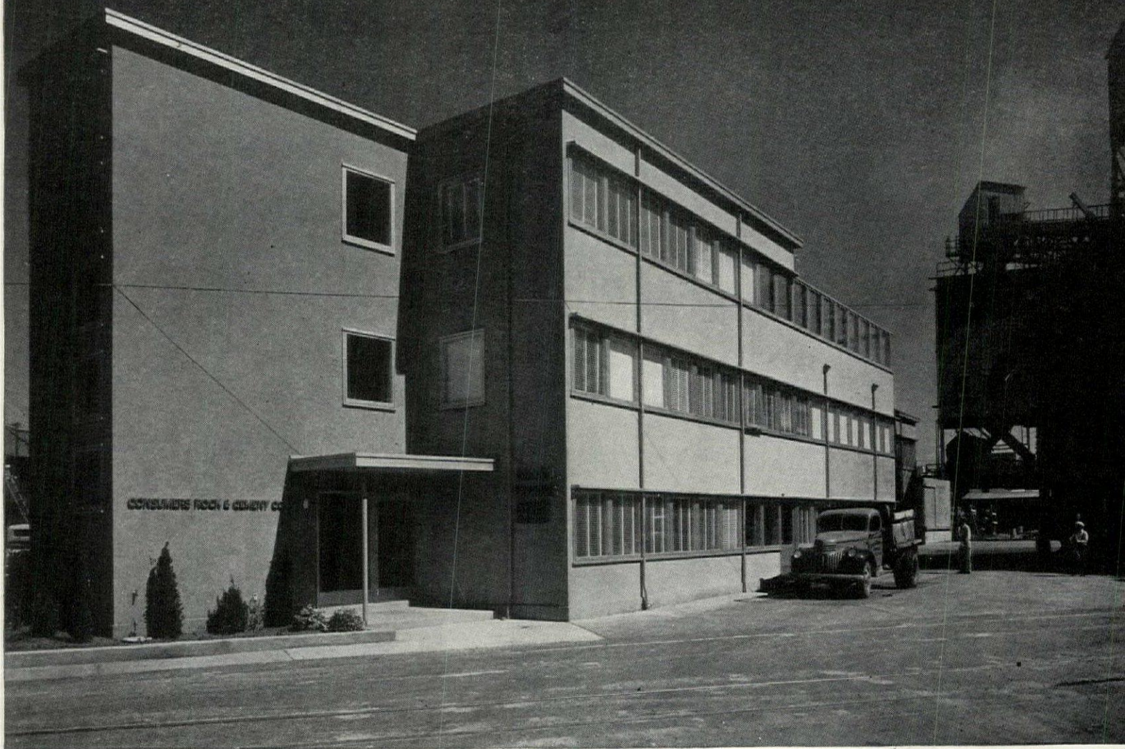
EXTERIORS ARE BRUSHCOATED BLUE-GREY, SIGNS AND COLUMN AT ENTRY ARE CORAL AND ALL TRIM IS PAINTED ALUMINUM
