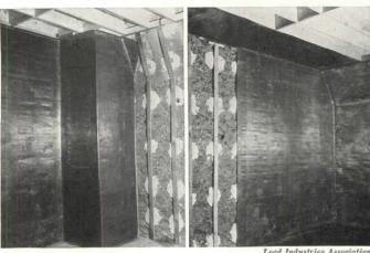
Laboratory sound insulation employing 4 lb. sheet lead on wood furring strips, seams soldered. Finish, fibre board on lead chairs.
