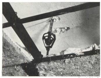
RESILIENT CEILING CONSTRUCTION: Holmes System of Sound Insulation. This construction employs a spring to absorb vibration. On top of the metal lath is a layer of sound absorbing material.
