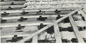
**"FLOATED" FLOORS:** Upper, floor floated on Cabot's "Quilt," Samuel Cabot Inc., Boston, Mass.; lower, floor supports resting on J-M Floor Chairs, Johns-Manville.
