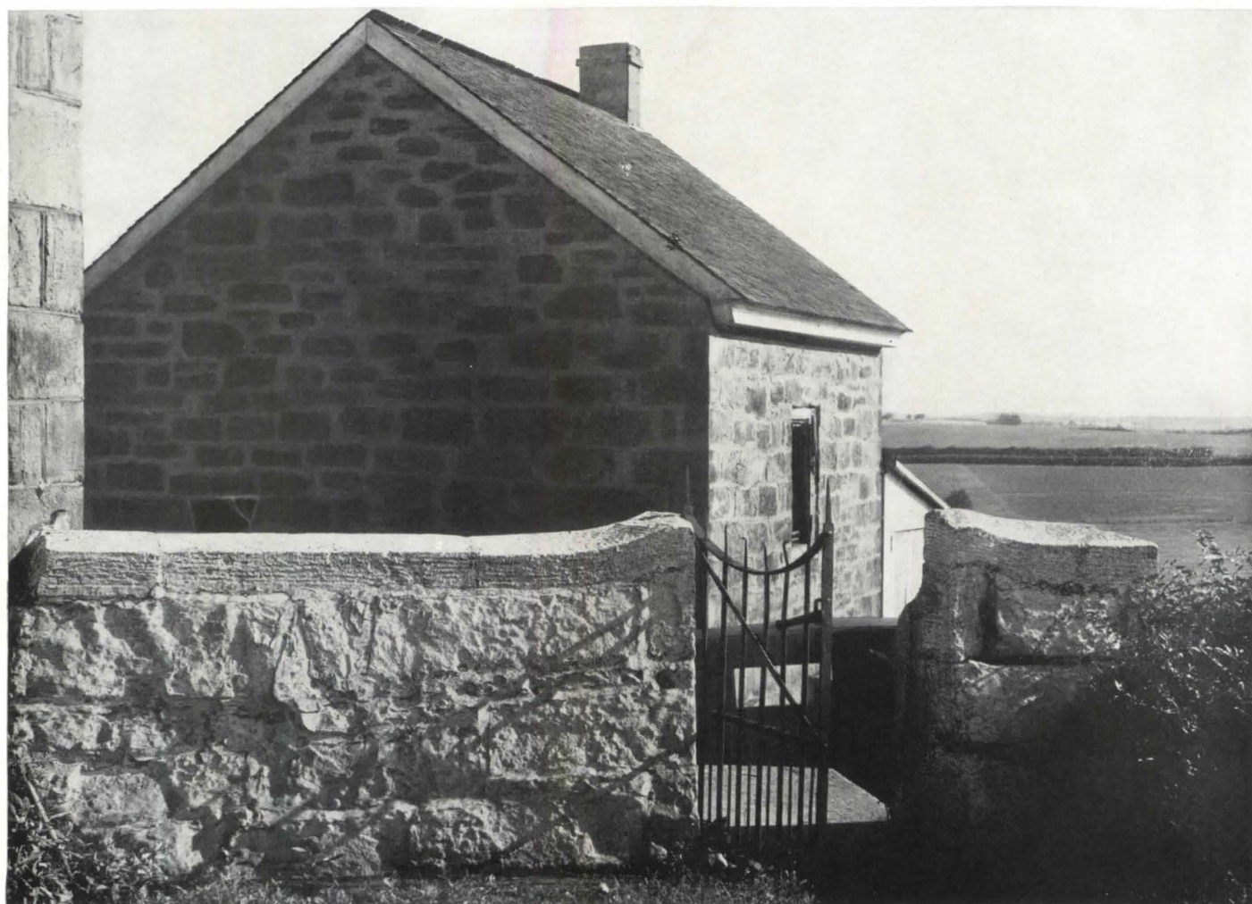
SOUTH SERVICE BUILDING
