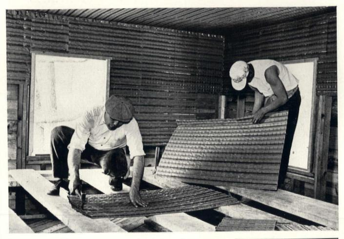
REYNOLDS ECOD FABRIC plaster base for the first time offers builders a basic product in two forms to meet all wall specifications—Metallated\* for outside walls, plain for partitions.
