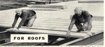
EASY TO USE. No detailed specifications needed with Gypsteel PLANK. It's light, dry, clean. And can be cut, sawed, nailed or bored as readily as lumber.
