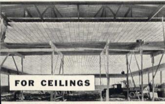
TULL FIREPROOF RATING. Gypsteel PLANK gives flat ceiling construction with maximum fire protection to supporting teel. Especially recommended for ceilings in garages, audioriums, theatres, etc. Saves heat loss, lowers insurance costs.
