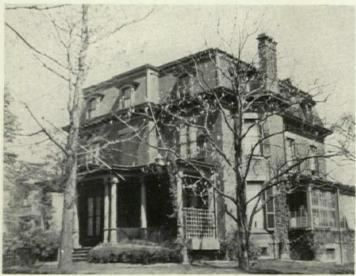
The original mansard roof of bad design has been cleverly wiped out by masking it with an attic treatment above the cornice that comes around and "ties in" to the new portico. A splendid solution which should prove heartening to the myriad victims of full-blown Victorianism.
