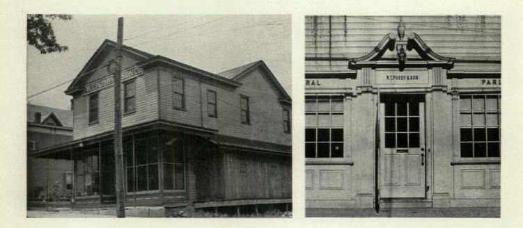
A most happy remodeling and modernizing of an unsavory, rundown, old building into a clean bright adaptation of Colonial design. The pediment triangle formed by the roof was completed by carrying the cornice across the facade, and adding a pilaster at each side. The vicious porch shed was removed, a new door and windows, a new terrace and steps built. Some new paint completed the magic on this exterior.
