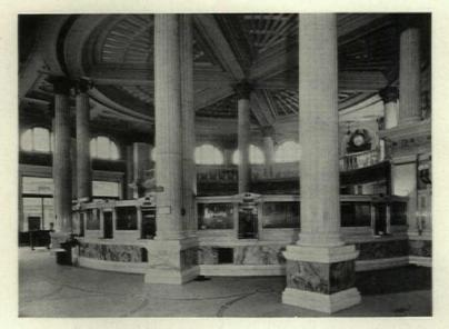
The former banking room was three steps above the sidewalk, and arranged on an old fashioned circular plan as shown below. The alteration lowered the floors to the street level, and extended the bank space to include the entire first floor of the office building. Eight old columns were eliminated, and seven new ones added, in new positions. The alteration now provides the bank with growth reserve facilities for an estimated period of twenty-five years.
