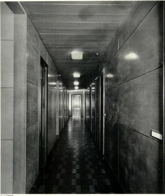
One of the few places in the offices where transite may be seen in the raw, a typical office corridor. Not even paint has been used to cover the dull gray of the finished sheets, the joints of which are marked by chrome beads. The same acoustic tile, but not in 12 x 12 in. units, is used for the ceiling, which has been dropped 18 in. to conceal the air conditioning ducts. The flooring here is asphalt tile
