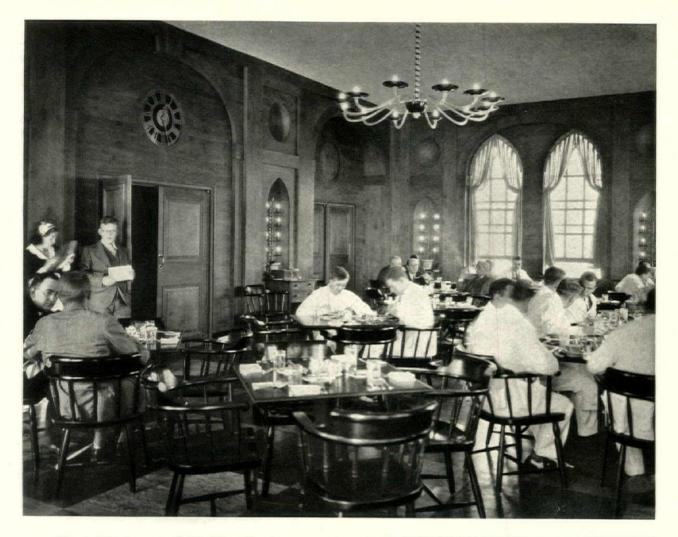
The staff dining room, finished from floor to ceiling in American white oak selected as to grain and knots. Black-and-gold and gray rubber tile, 36 in. square, is used for the floor, and the ceiling is of acoustic plaster. The chairs were designed by the architects for general use throughout the hospital. The chandelier is of white and purple glass, and the candelabra in the niches are from an old Sicilian model
