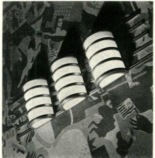
Lighting fixtures in the RKO Roxy Theater in Rockefeller Center. The frosted glass panel in the soffit of the auditorium balcony, right; one of the indirect units for the mezzanine walls and staircases, below left; frosted glass ceiling unit in the principal lounge
