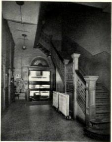
The entrances to the offices and studios in Carnegie Hall, New York, modernized by Edward I. Shire. Without disturbing the old structure or finish, the corridors were remodeled by using metal furring and cement plaster. New doors, radiators, light fixtures were also installed
