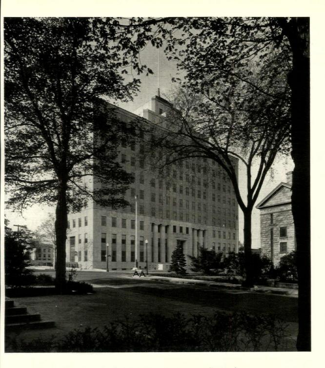
The county office building is becoming a necessary adjunct to the efficient conduct of county affairs. Federal financial aid is made available through the N.R.A. for such needed buildings. The exterior facing of this structure is brick, granite and limestone. It was built at a cost of about 54 cents a cubic foot
