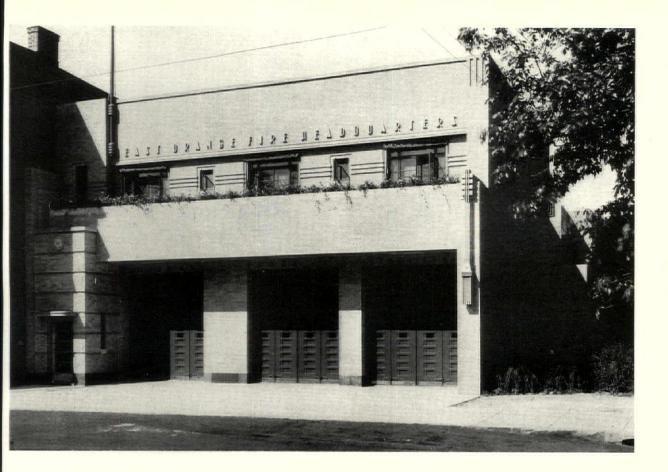
The design of this suburban fire station suggests modern Swedish architecture in its severe lines and simple detail. Faced with light tan brick, the building is of fireproof construction, with brick bearing walls, steel and concrete floor construction and pile foundations. Copings and sills are sandstone, base red granite, and all exterior metal trim green bronze
