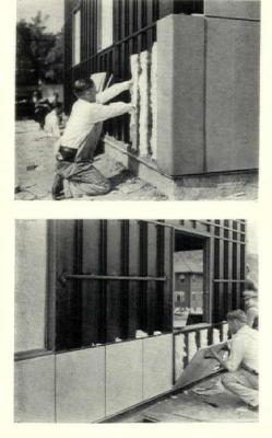
Left and around: the exterior panels are screwed onto the Wheeling steel house. The screws are applied to furring channels welded to the wall section and washers bear on panel flange. At the right is a view of the sub-floor, the bottoms of the channels resembling the usual two-by-eights. And at the lower right, Wheeling steel studs accommodate Wheeling plumbing and a Wheeling conduit.
