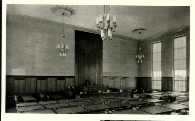
The board of supervisors room is simply treated with artificial stone walls above a dado of Brazilian Hud oak. The ceiling is plaster. Ventilating diffusers are combined with the lighting fixture shields
