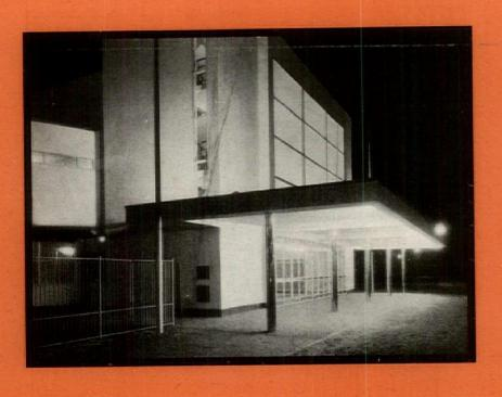
The whole building is built round a skeleton of reinforced concrete with white cement rendering. At the main entrance, here illustrated, the columns which support the fence-roof are of reinforced concrete sheathed in stainless steel.
