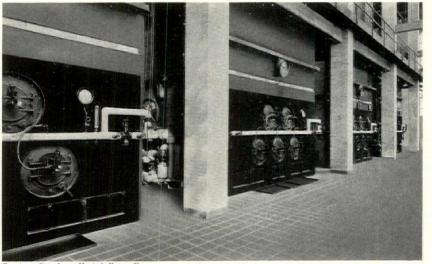
The battery of oil-fed boilers each rated at 1,600 hp. The electric control apparatus regulates oil feed, speed of forced draft fans, quantity of air supply and of stack gases
