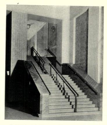
Marble staircase leading to second floor shops of the arcade. Fluted marble pilasters repeat the vertical motif of the exterior, and the coloring of the marble walls is blended with the terrazzo mosaic floor. All trim, including stair rails, is while bronze, as are the bracket fixtures
