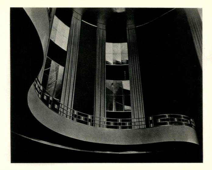
Looking upward loward the mezzanine balconies surrounding the grand foyer. The walls are covered with a washable wall fabric, broken up by silver mirrors, and golden brown drapes. The balcony facing is painted to match, and the railing is of bronze and nickel bronze. The doors leading from the ticket lobby and into the auditorium are of stainless steel with bronze plaques. On the page opposite are the ground floor and first mezzanine plans, and the section
