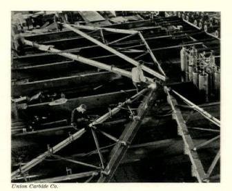
A view in the shop, showing assemblage of a large truss and joining of the members by oxyacetylene welding
