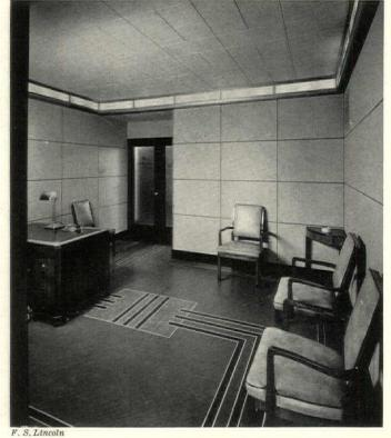
Ninth floor reception room, inlaid asphalt tile flooring, fabricona wall finish, with beads painted black, and acoustic tile ceiling
