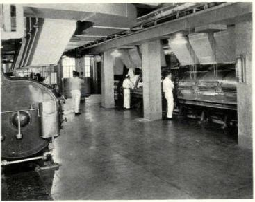
The modern laundry equipment installation provides sorting-room hoppers above the battery of washing machines, providing direct chutes and hoppers to the proper machines
