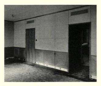
Steps one, two, and three in the erection of the partitions. No. 1 (at top) shows the study set up over the finish flooring, with electric conduits running through the base. No. 2 (center) shows the dado secured to the study; and No. 3 (above) the wall sheets erected ready for snapping the base into position. The entire operation can be accomplished in a few hours
