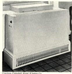
Unit air conditioner which contains silencer as well as filter
