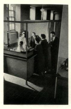
Registration desk of the out patients' department (above) which has a "greengranite" 1 in. ceramic tile dado, with hand finished plaster flush with tile above, and a floor and base of red quarry tile
