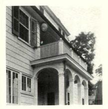
Typical garden floodlighting, above; at left, the lighting unit under the eaves which supplied the illumination
