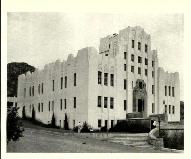
Picturesquely located in a canyon this building has a vigorous verticality. Of reenforced concrete bearing walls with a plastered finish and an interior construction of steel framing, it cost \$275,000. Ornamental metal work is of bronze, the roof of copper. Placer miners are shown over the main entrance, below
