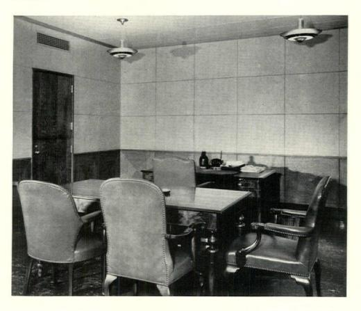
In this office the walls are finished in fabricona homespun, and the dado is oak veneer. Above the dado the joints are butted. No carpeting is used over the asphalt tile flooring
