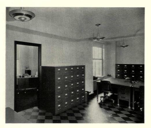
Above, an office suite finished in fabricona with taku veneer for the dado. Below, typical clerical office which has an asphalt tile floor, painted transite walls and acoustic tile ceiling
