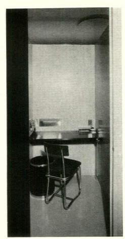
IN THE vault lobby above, the floor is beige rubber tile, the 7-foot high wainscot is black marble, and the wall above it is plaster, painted a dead white. The exterior of the vault is yellow bronze except around the door which is stainless steel, as is the casing of the round column. In the coupon lobby below the columns are faced with a dark brown rubber tile
