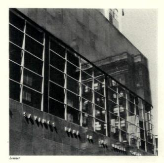
An exterior view of the 23-foot high banking room window detailed on the opposite page. Note the apparent lightness and pattern of the horizontal and vertical aluminum mullions
