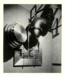
Above is the conditioned air supply to the vault. It may be removed at will. Below is a typical fan supplying one of the main ducts
