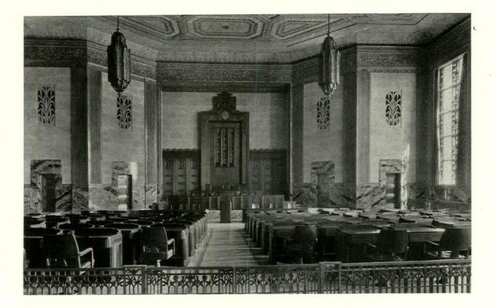
Three views of the House of Representatives. The keynote of color is derived from the Jaune Benou marble used for the wainscot and trim. The fluted pilasters are of polished Sienna travertine, with walls of light pink Crazannes Anteor stone. The floor is of Roman travertine, bordered and paneled with marbles. Desks and chairs are of Australian laurel, upholstered in blue leather. The basic lighting is indirect, but visible fixtures and other metal work are bronze
