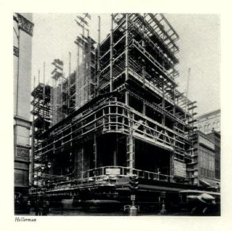
A progress photograph of the building showing the trusses behind the supports of the granite facing above the banking room window, the east wall columns and the cantilevers
