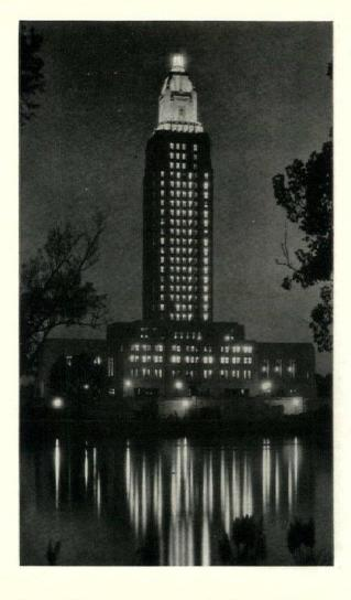
The building was erected by the George A. Fuller Co. in a year's time from the laying of the foundations in January, 1931. The building rests on a foundation of some 1,900 reinforced concrete piles 16 in. square, averaging in length between 40 and 60 ft., each designed for a 50-ton load.
