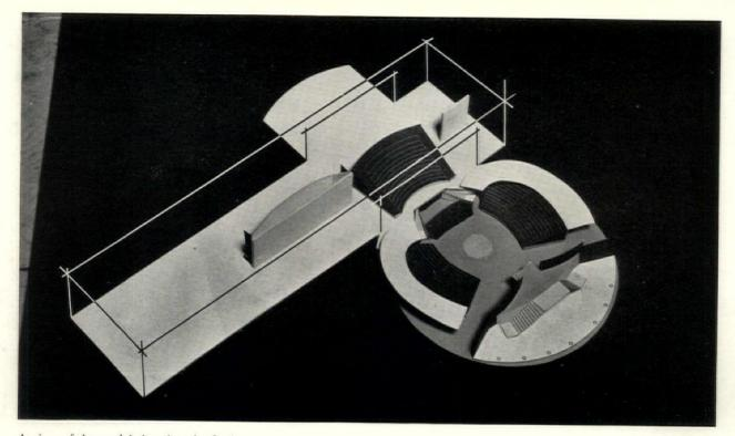
A view of the model showing the flexible enlargement possibilities when used as an arena, the movable seats of the smaller auditorium having been rolled across to augment the seating capacity of the main auditorium. The cyclorama has been moved to its storage position
