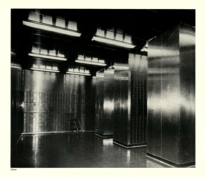
A NEW type of design employing extremely thin walls has made possible the vault location on the third mezzanine with but few special structural provisions. The interior finish is stainless steel, with fittings of bronze and lettering in vermilion red. The floor is dark blue rubber tile. Maximum protection is afforded by means of automatic radio and special electric devices. It is noteworthy that the architects checked every detail of the design as it
