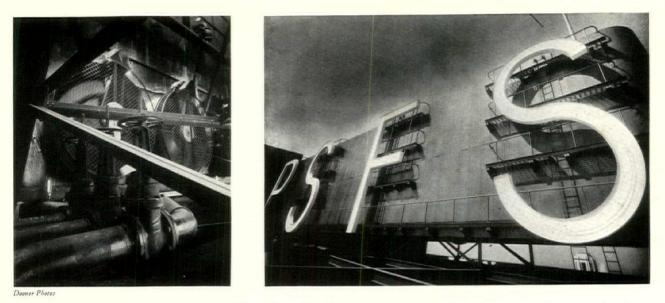
The steel background for the huge electric sign on the roof of the office portion of the building conceals part of the air conditioning equipment shown at the left. The letters of the sign are 27 ft. high and 15 ft. wide. They are formed with a white porcelain enamel face and are lighted by red neon tubes. The background of the sign is painted a cobalt blue
