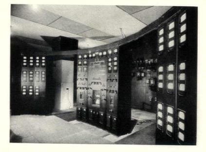
At the left is a view of the main bus connections for the electrical system in the sub-basement. At the right is illustrated the board from which all feeder switches, transfer equipment and emergency switches are controlled
