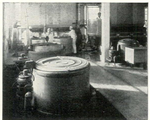
The washroom in the new laundry, machined with mass-handling "American" equipment—easily handling many more tons of work daily, in 9 hours instead of 16.
