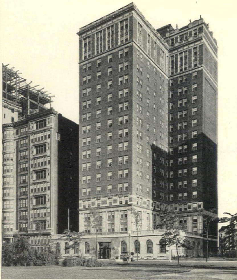
JOB 1108—APARTMENT BUILDING—CHICAGO, ILL. GEN. CONTRACTOR—McLENNAN CONSTR. COMPANY—588 PILES—9,549 FEET Architect: FUGARD & KNAPP
