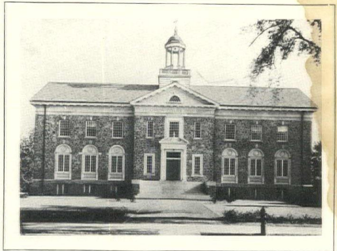
Dickinson College Gymnasium makes certain of adequate light at all times. It is equipped with an Exide Emergency Lighting Battery System. Wm. W. Emmart, Baltimore, Architect.
