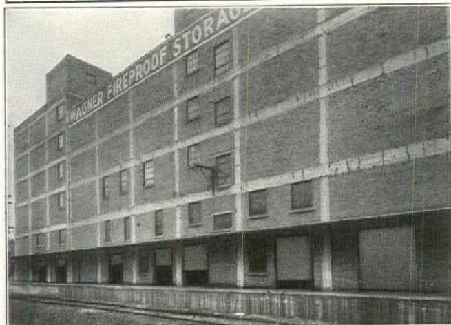
KINNEAR INSTALLATION—WAGNER FIREPROOF STORAGE & TRUCK CO.
