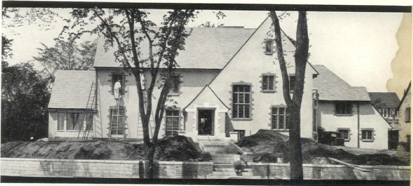
Provision is made for telephone convenience in the residence of Mr. J. R. Stewart, 2424 West Lake of the Isles Boulevard, Minneapolis, Minnesota, by built-in conduit serving six telephone outlets, including one in the basement game room. CARL A. GAGE, Architect, Minneapolis.
