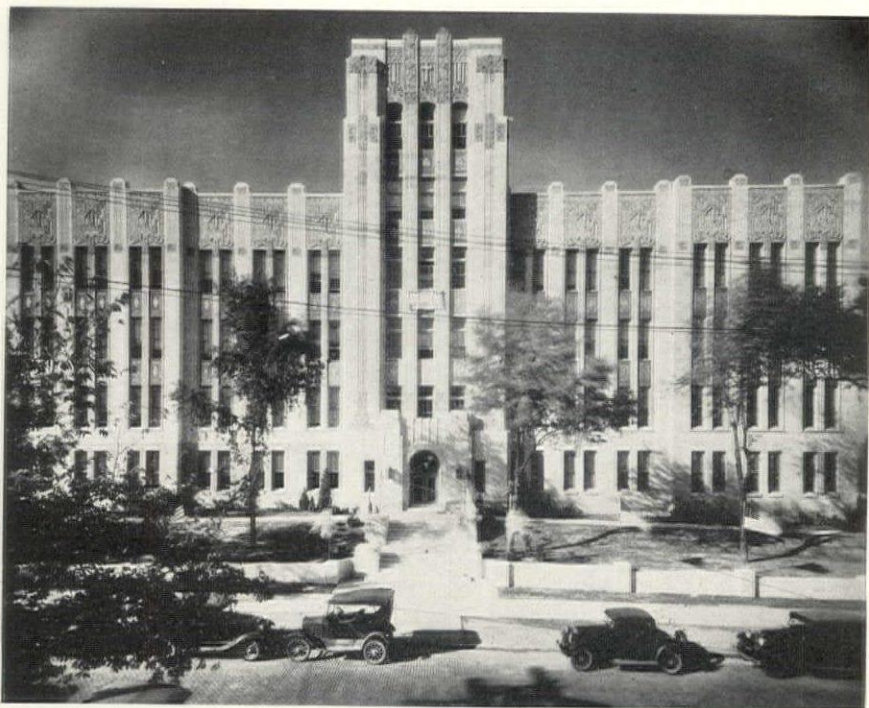
The Faculty and Administration Building at Creighton University; Leo A. Daley, Architect. The building is of fireproof construction, with aluminum spandrels and a limestone facing
