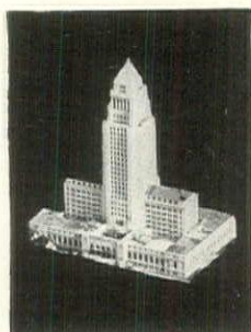
City Hall, Los Angeles, Cal. Omicron-protected terrace floors. . . Parkinson, Martin & Austin, Architects.
