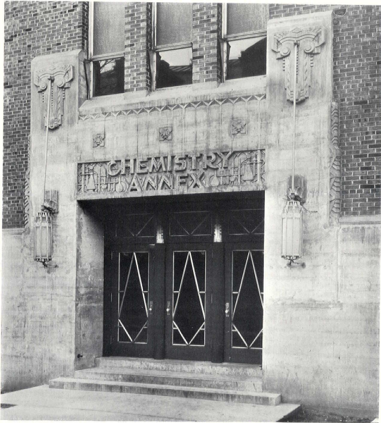
The entrance to this building is entirely of concrete. Plaster moulds of the ornament were set in the wood forms and the regular concrete mix was used throughout
