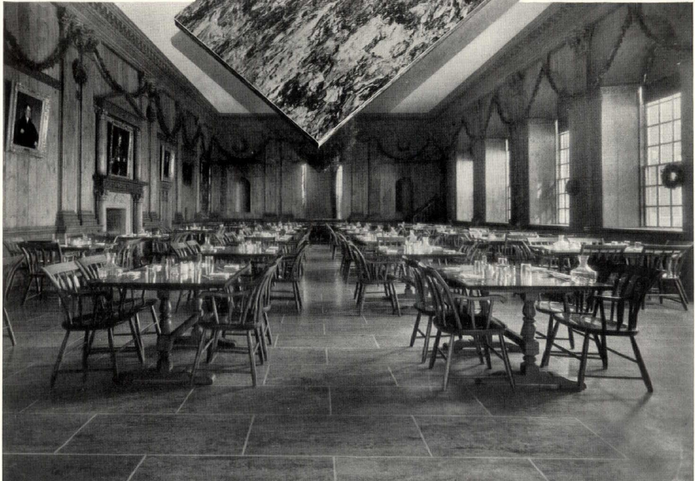
Dunster House at Harvard University. Coolidge, Shepley, Bulfinch & Abbott, Architects. In the Dining Hall, shown below, the Stedman Rubber Floor is laid in rectangles of O.S. Red with interliners of Plain White.
