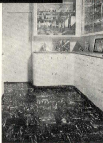
Goodyear Rubber Flooring as laid for apartment pantry — 1301 Astor Street, Chicago — Philip B. Maher, Architect
