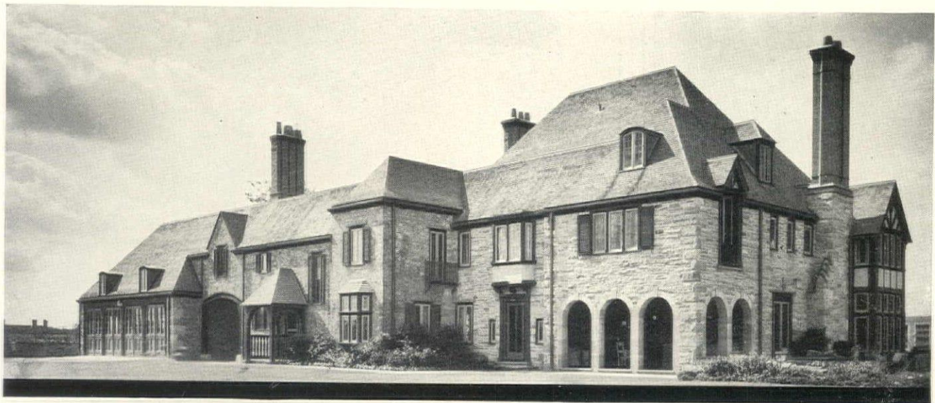
Built-in conduit and nine outlets provide for telephone convenience in the residence of Mr. Wilbert J. Austin, Sherbrooke Road, Shaker Heights, Cleveland, Ohio. MAIER & WALSH, Architects, Cleveland
