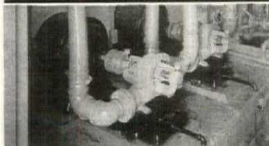
A Model 6F6 with 7½ h.p. motor delivers 100 g.p.m. at 125 ft. in this building at 91st St. and Riverside Drive in New York City.
