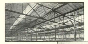
Bendix Aviation Building, South Bend, Indiana. Below—roof deck *ready for composition cover-*ing. The entire roof of Featherweight slabs was erected in winter—an area of over 300,000 sq.ft. And this expanse represents but half the area of Federal roofs in use by this company!
