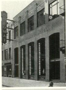
Passers-by are attracted by the unusual exterior illumination—lighted panels installed at the sides of the window jambs.
