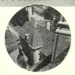
In this structure, the floors and walls—interior and exterior—are of reinforced monolithic concrete. The exterior has no finishing coat—the concrete was purposely left just as it came from the forms. Structural frame is of steel. Exterior ornamentation was cast in place. So built, this edifice offers positive assurance of firesafety and long life, with little if any structural maintenance through the years.
