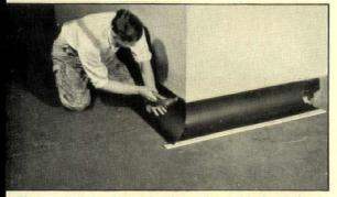
Here we see the mechanic fixing the cove-base and border in place by means of headless brads, placed on 3'' centers, 1/4'' below top of base.
