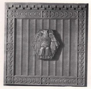
In color, aluminum resembles silver, but with a slightly bluish tint. On weathering, the color becomes darker. This is due in part to the protective coating of oxide which forms on the surface, and to the accumulation of foreign particles from the atmosphere. A polished surface will remain bright much longer than a rough or "as cast" surface, since the dust and dirt in the air can not collect on it as easily.
