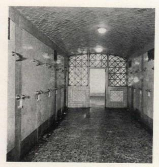
Men's Shower Room Showing Drain Gutter at Wall; Valves at Right of Shower Heads
