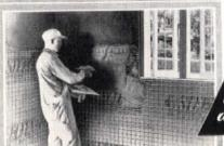
Ribbed STEELTEX reinforces plaster, insulates against heat and cold... deadens sound
