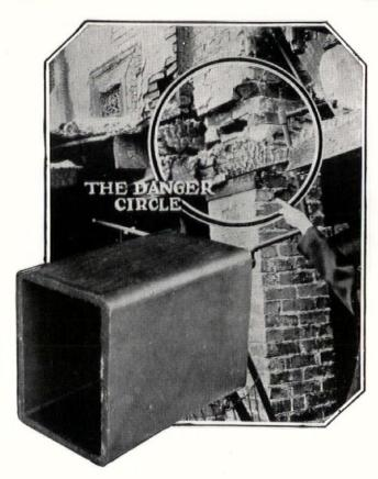
No more chimney fires when every house is built with fire clay flue lining
