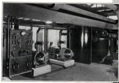
Equipment-Shone Duplex Ejector, Capacity 600 g.p.m.
