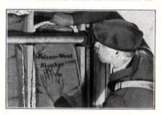
IT TUCKS IN! Balsam - Wool combines the highest insulating efficiency ever attained in practical house insulation with the important advantage of flexibility. In these two respects it meets squarely the requirements of true house insulation
