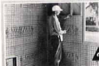
Ribbed STEELTEX is nailed directly to studs. Walls and ceilings are completely Blanketed
