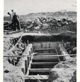
Left. Building the Walls of the Reinforced Concrete Septic Tank and Siphon Chamber
