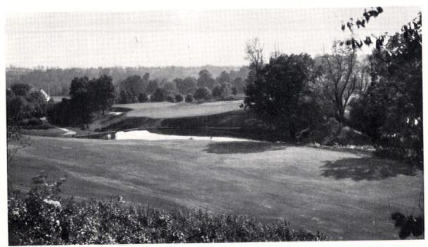
The 18th Hole at the Knollwood Golf Club, Near White Plains, N. Y., Taken from the 200-Yard Mark. The Fairway in the Foreground Was Swampy and Required an Extensive Drainage System. The Fairway Across the Pond, in Front of the Green, Was a Steep, Unplayable Slope Which Had to be Graded by Making a Cut on the Right and a Fill on the Left. The Green Itself is on a Location Formerly Occupied by a Rubbish Heap and an Old Greenhouse Foundation. The Construction Was Heavy, but the Hole Appears Natural
