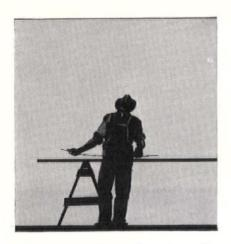
The expert workman takes a foot rule, measures the distance, and cuts the pipe to fit the space where it is to go.
