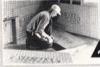
Ribbed STEELTEX is readily cut ... and shaped to fit around window and door openings
