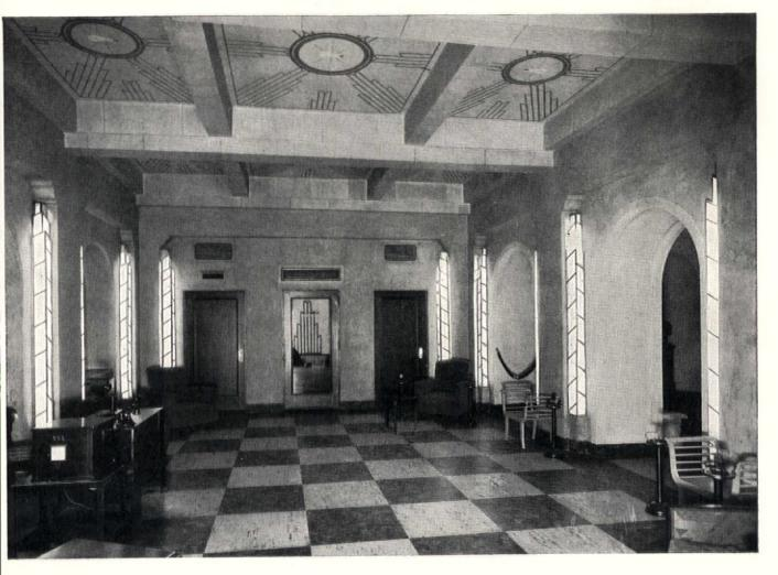
Illumination in this reception room of the Westinghouse Lamp Company's exhibit comes from the Frink illuminated pilasters...The "Solite" glass is evenly illuminated by two vertical rows of Linolite Lamps, particularly well suited for this work because of their continuous filament.
