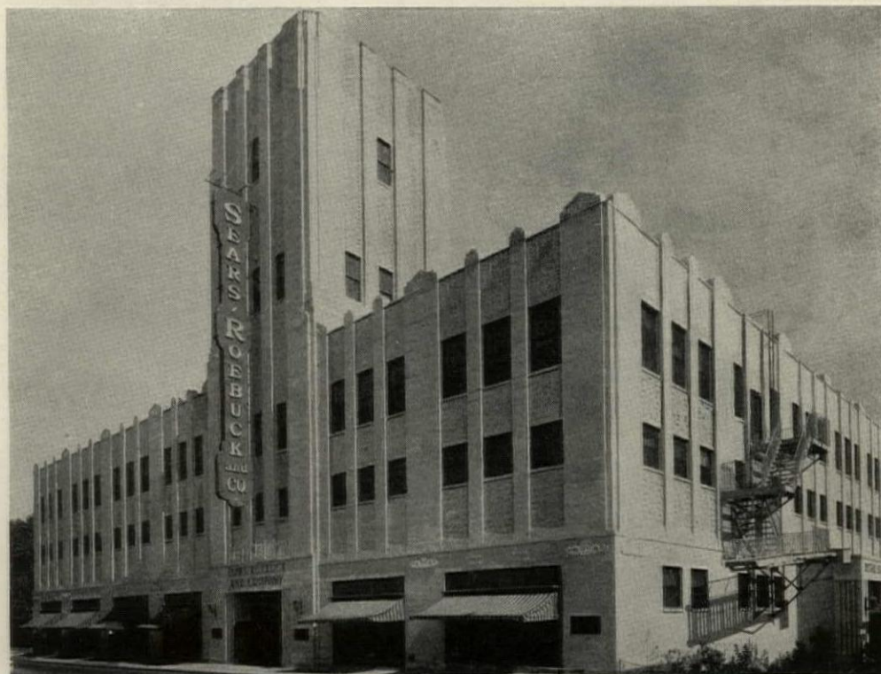
SEARS ROEBUCK BLDG., Cincinnati Architects: Nimmons, Carr & Wright Contractors: Westlake Constr'n Co.
