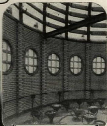
Interior floodlights inside dome, 34th floor
