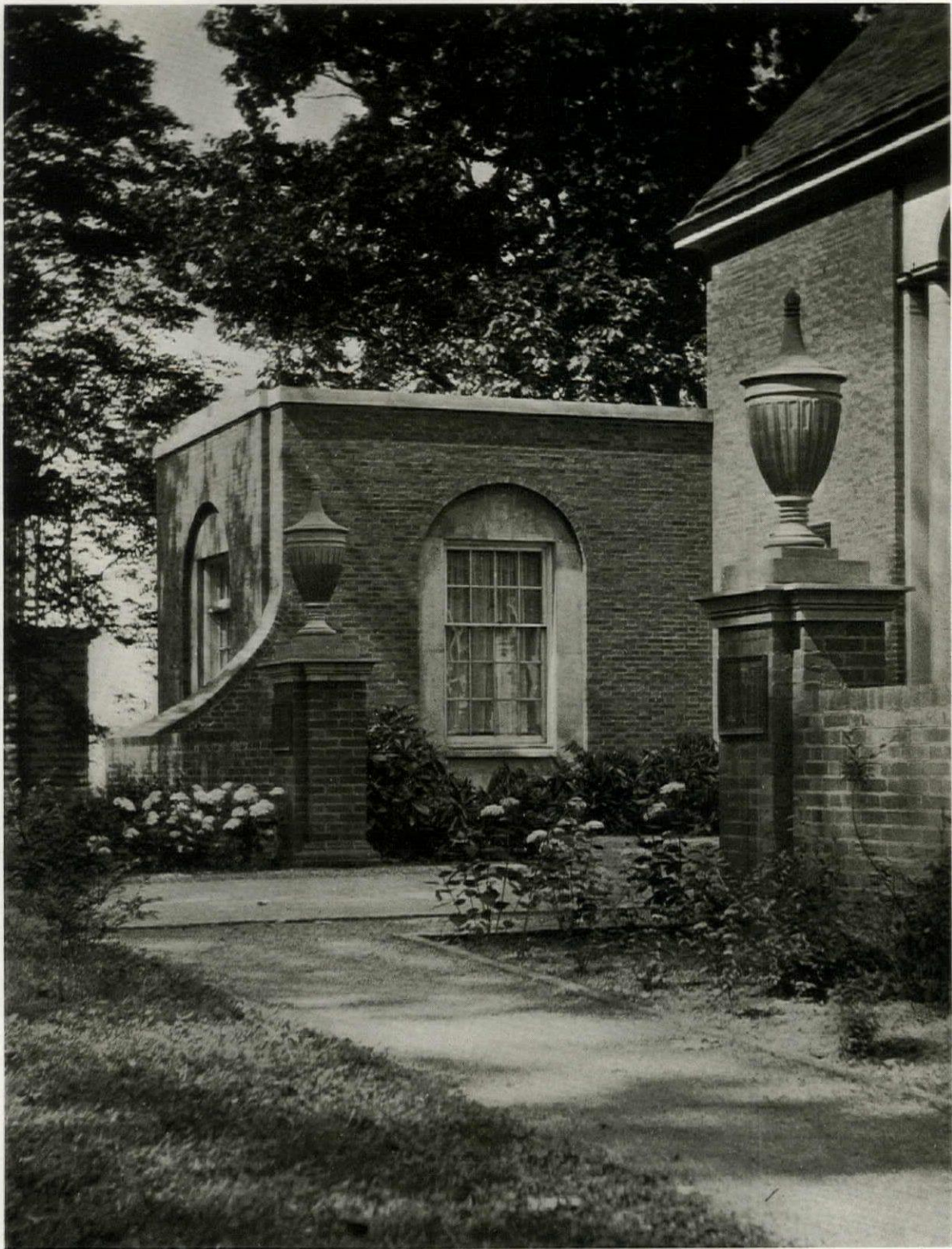
DETAIL OF THE ENTRANCE COURT WOMEN'S PHYSICAL EDUCATION BUILDING WEST VIRGINIA UNIVERSITY, MORGANTOWN DAVIS, DUNLAP & BARNEY, ARCHITECTS
