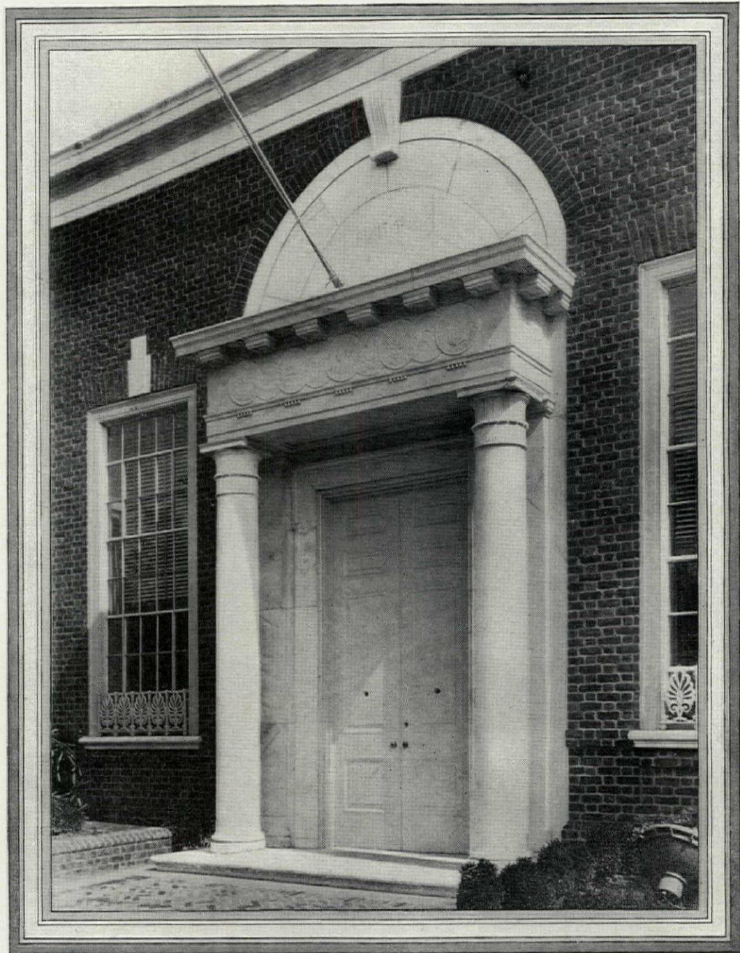
MAIN DOORWAY — HOLMESBURG TRUST CO., HOLMESBURG, PA. DAVIS, DUNLAP & BARNEY, ARCHITECTS
