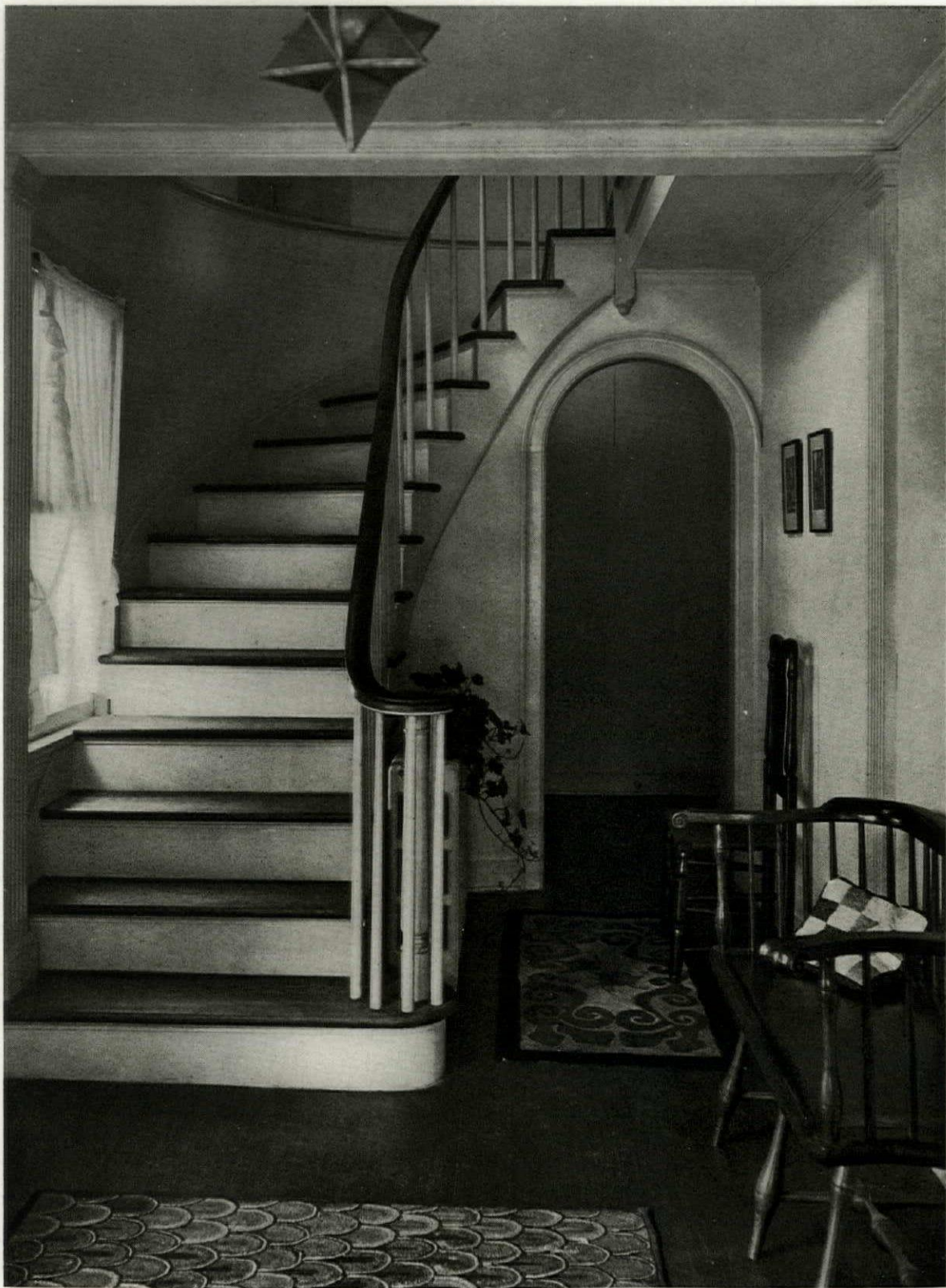
STAIR HALL, EARLY AMERICAN FARM HOUSE, EASTCHESTER, N. Y. JAMES JENNINGS BEVAN ARCHITECT AND OWNER
