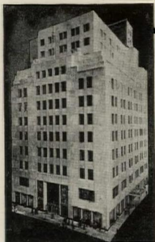
Roofed with A T P STEWART AND COMPANY BLDG., 721 Fifth Avenue New York City Architect: Warren and Wetmore General Contractor: Caldwell Wingate Company Roofing Contr: Jacob Ringle and Son
