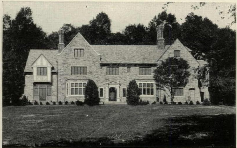
In the residence of Mr. Philip N. Lawes, 56 Highland Avenue, Montclair, N. J., there are ten telephone outlets, including one in the garage and one in the basement. Conduit built into the walls and floors conceals the telephone wiring. W. LESLIE WALKER, Architect, New York City.
