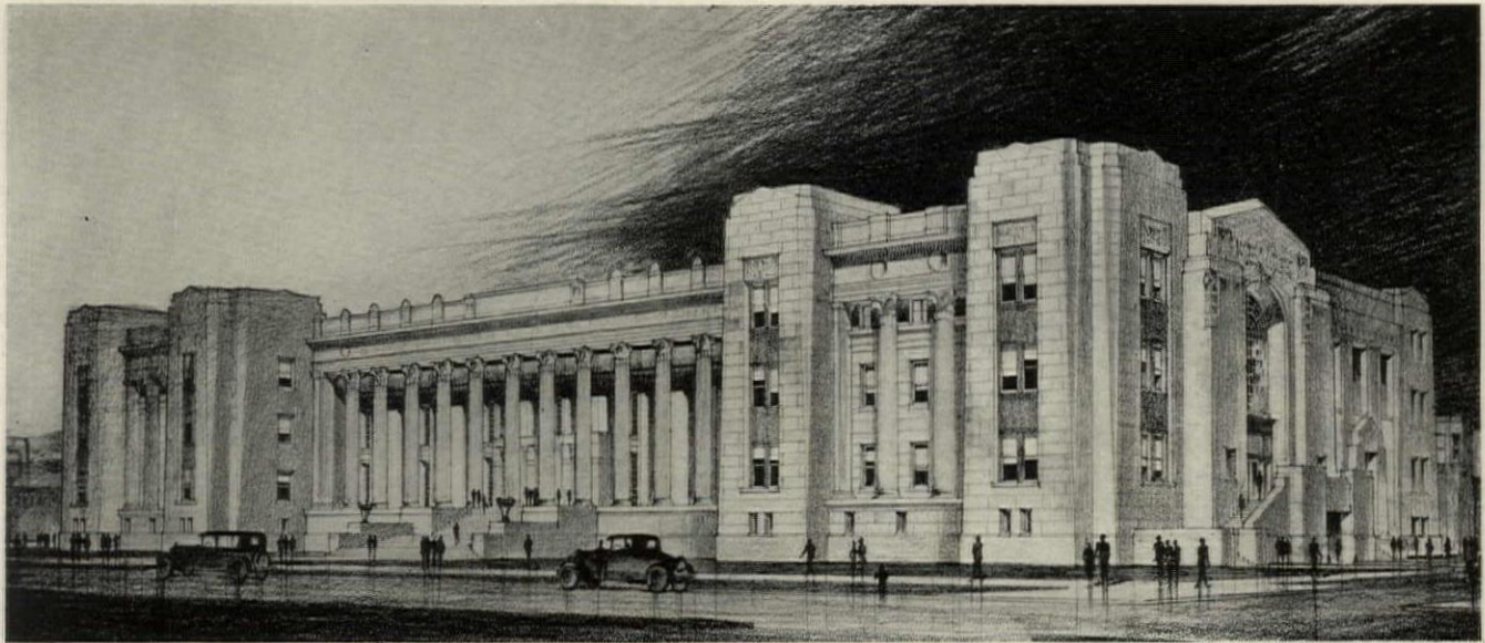
Criminal Courts and Jail Building at New Orleans, La. Equipped with Douglas Plumbing Fixtures and Solid Nickel Silver Trimmings. Diboll & Owen, Ltd., Architects. E. A. Christy, Associate Architect. James M. Todd, Mechanical Engr. Sciambra & Masino, Inc., Plumbers
