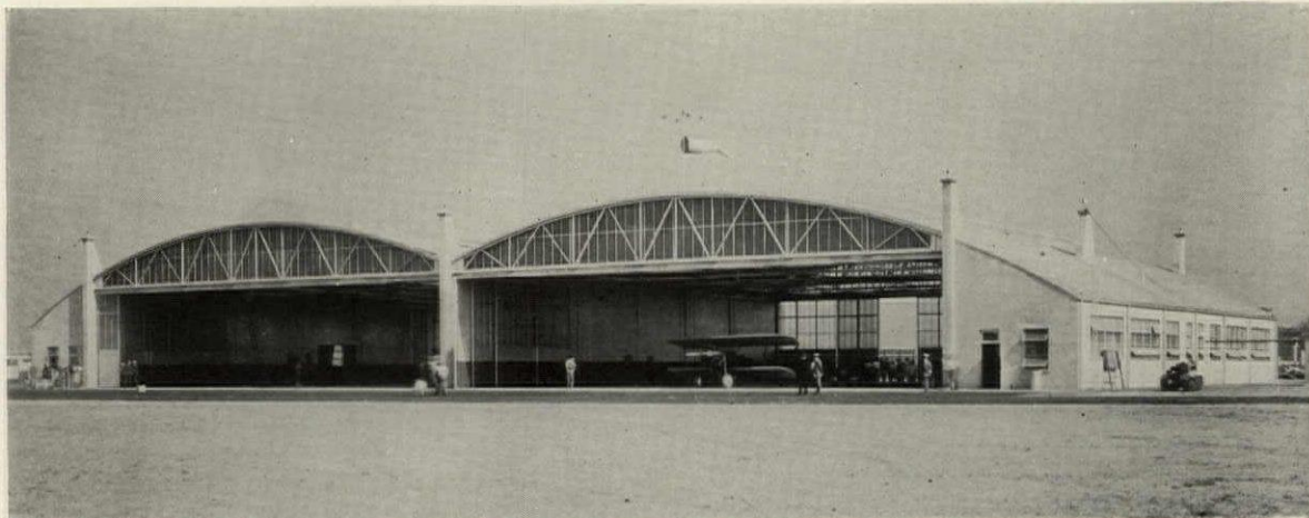
Fireproof Hangars at the Central Airport, Camden, N. J., Fifteen Minutes From the Center of Philadelphia
