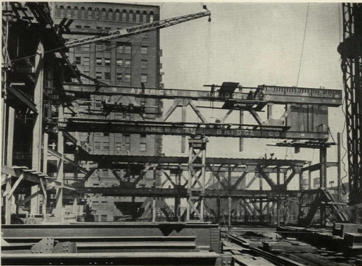
Trusses of the North Wing Over the Railroad Tracks
