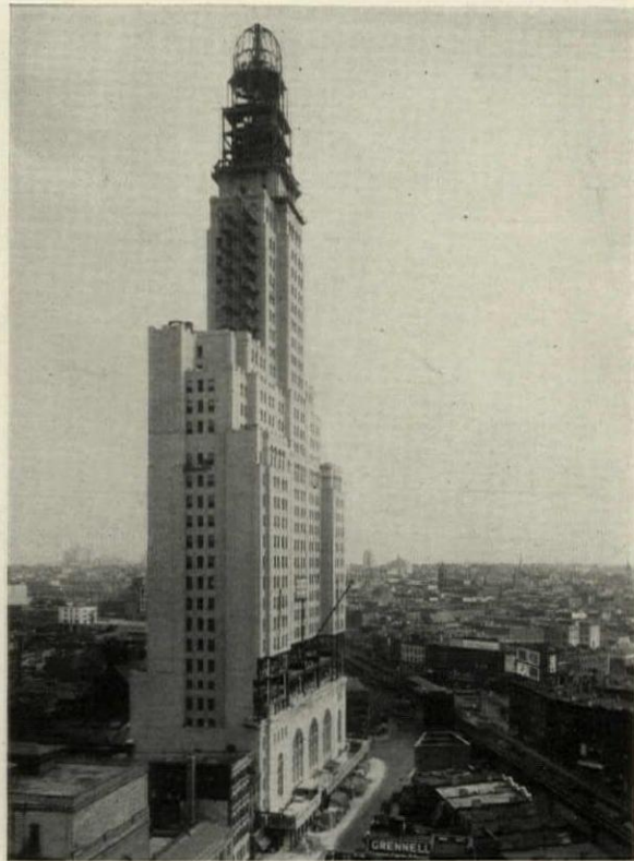
General View, Williamsburg Savings Bank Building, Brooklyn
