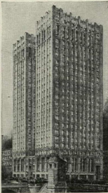
1130 Sarco Radiator Traps in the Engineering Bldg., Chicago
