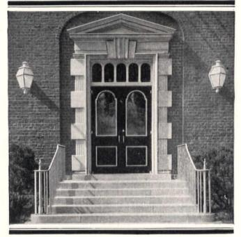
This door trim and the stair rails, fabricated from Aluminum alloy, reflect the spirit of modernism in the material employed.
