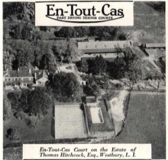
T HE dull red color harmonizes well with the landscaping, and the perfect playing surface is similar to fine turf. The imported surfacing material, made of a patented processed clay is laid over a resilient and quick-draining foundation. Since 1912 thousands have been in use in England and on the Continent, and they are rapidly becoming popular in the United States. A large per cent. of these are repeat orders.
